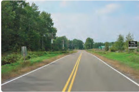
County A, Burnett County
