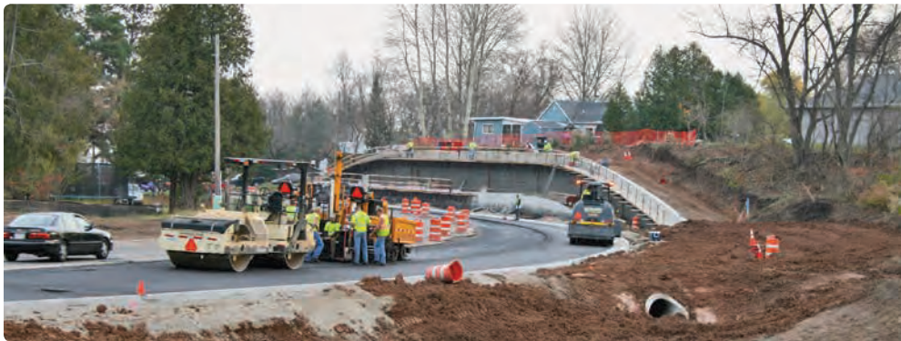
Work at the WIS 54 bridge over Duck Creek in Brown County
