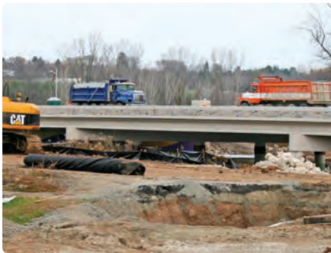
WIS 54 bridge, Brown County
