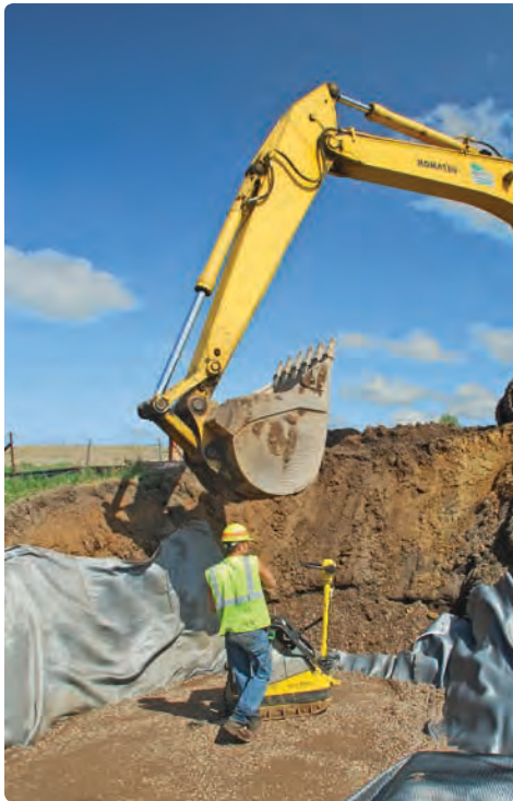
Hwy 40 bridge construction, Chippewa County
