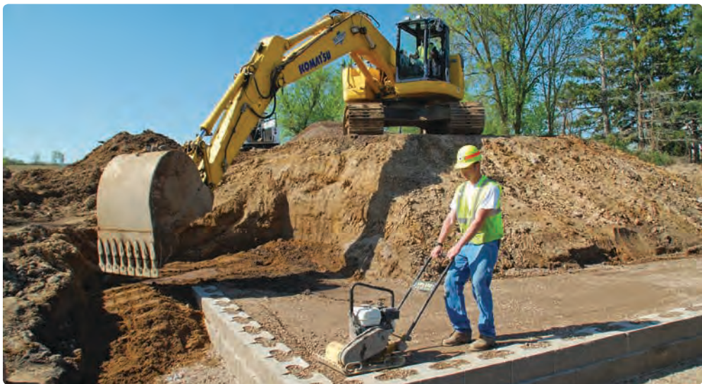
WIS 40, Chippewa County
