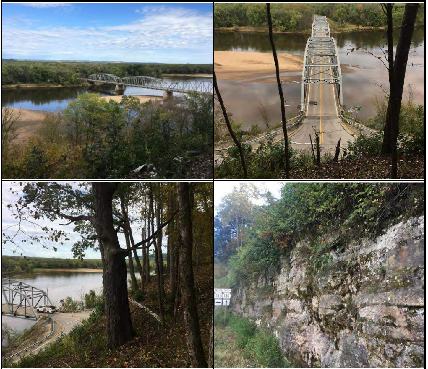
Figure 10. Wisconsin River Crossing and Bluff
