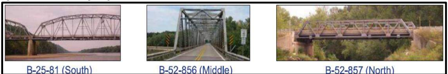
Figure 5. Photos of Existing Bridge Structures
