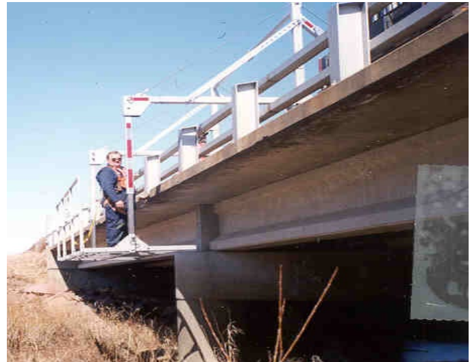
Class 9118 Scaffolding w/ electric hoist
