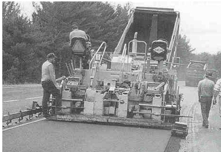
Class 712 Bituminous Equipment Self-propelled paver and finishing machine
