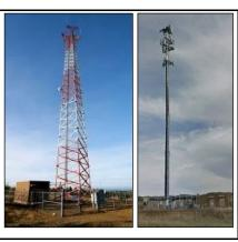
Macro cells may be installed on rooftops, building facades, monopoles and other steel structures. These cells provide coverage over a broad area (up to several miles). When on monopoles, they are typically over 50 feet in height.
