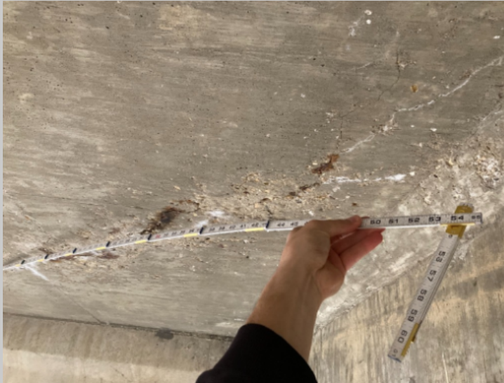
B-52-053, WIS 80 bridge over Pine River
