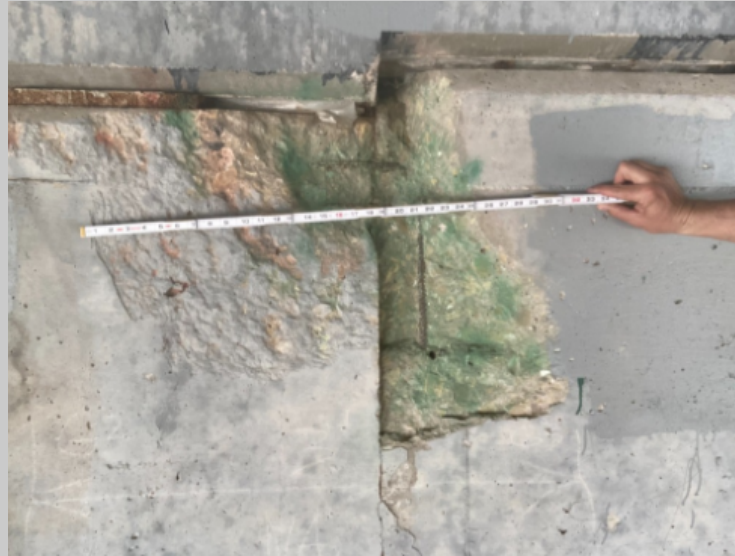
B-52-108, WIS 80 bridge over Pine River
