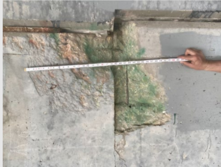
WIS 80 bridge over Pine River
