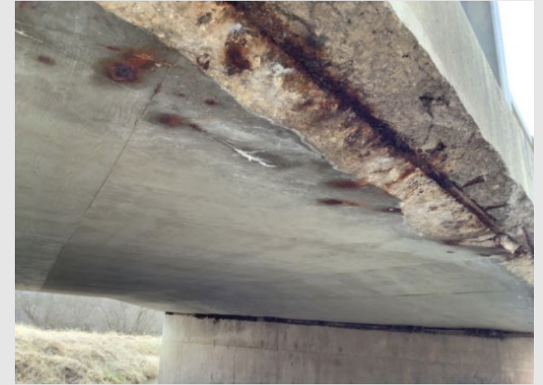
WIS 80 bridge over Pine River
