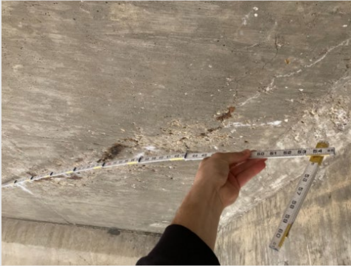
WIS 80 bridge over Pine River
