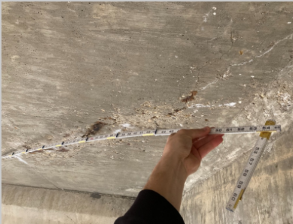
B-52-053, WIS 80 bridge over Pine River
