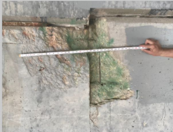
B-52-108, WIS 80 bridge over Pine River
