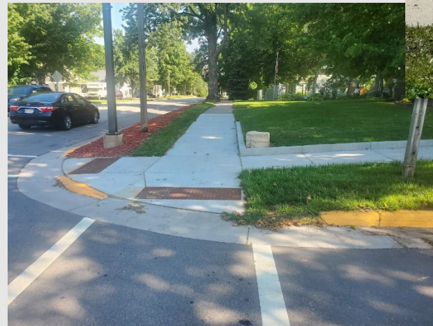
Example of an ADA compliant curb ramp
