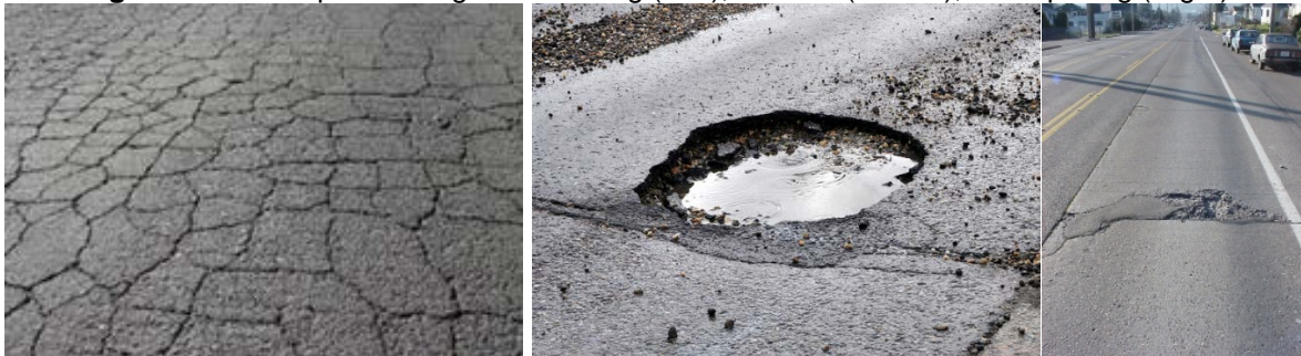
Figure 6-5: Examples of Alligator Cracking (Left), Pothole (Center), and Spalling (Right)
