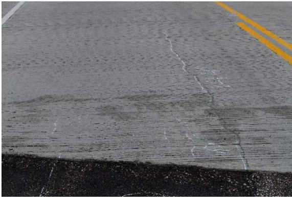
(a) A 12 ft long crack over the east abutment
