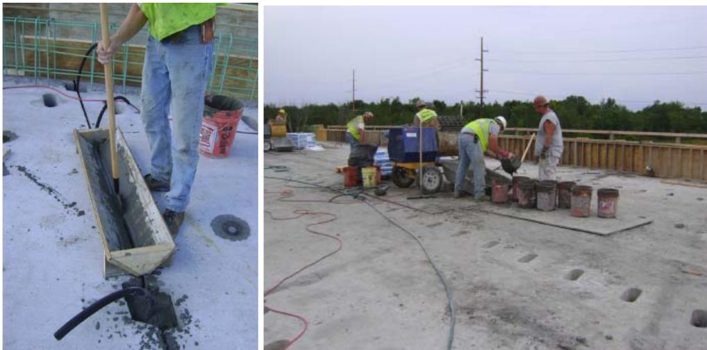
**Figure 2-13. Grouting of full-depth deck panel connections (Source: Courtesy of MDOT)**
