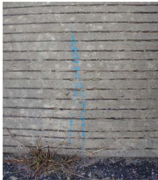
(b) A short crack over the abutment and above a shear key
