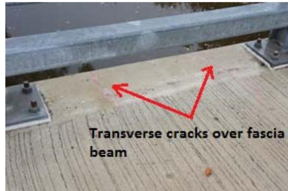
(ii) Transverse cracks over the fascia beam
