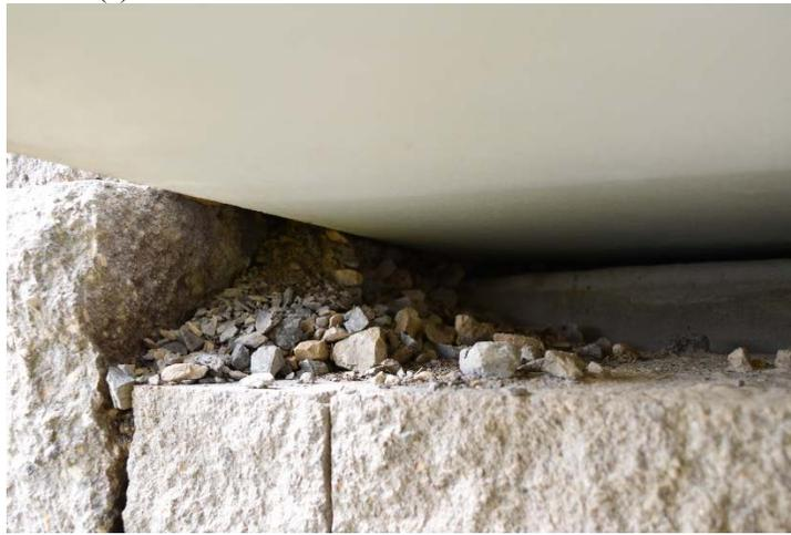
(b) Backfill material underneath the fascia beam
