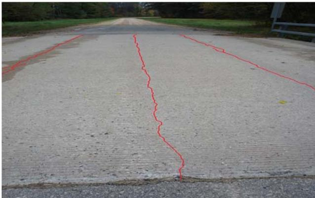
(a) Full-length reflective cracks
