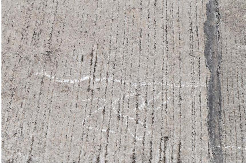
(a) Crack along the 4<sup>th</sup> shear key on west abutment
