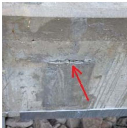
**Figure 4-12. A stress pocket exposed to surface water**
