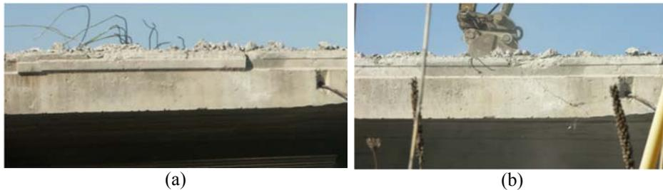
**Figure 2-6. (a) Shear key material attached to a beam and (b) beam surface after grout had fallen off**
