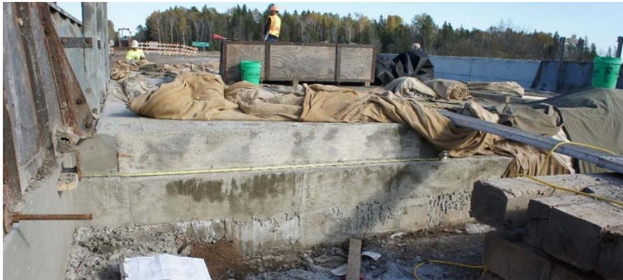
**Figure 5-2. Monolithically cast end diaphragm and deck slab**
