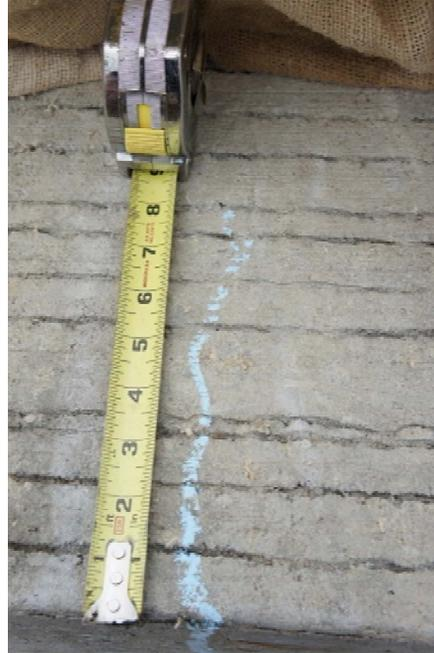
(b) Crack propagation along deck
