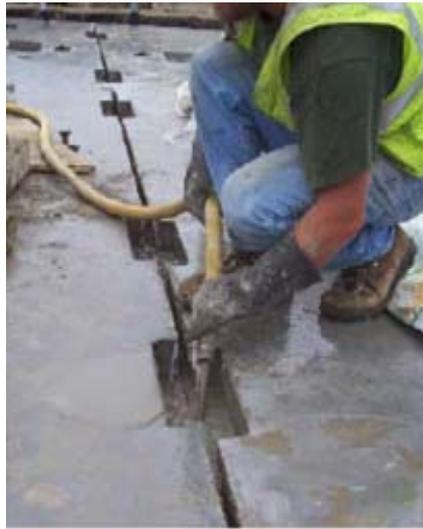
**Figure 2-12. Pumping W.R. Meadows Sealight CG-86 non-shrink grout (Source: Oliva et al. 2007)**
