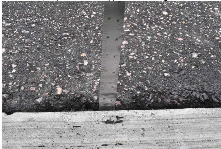
(b) Depth of the gap (3.5 in.) between the approach and bridge deck
