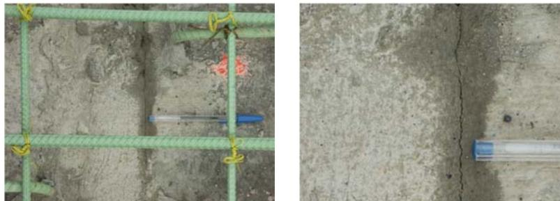
**Figure 2-7. Shear-key interface cracks before deck slab placement**
