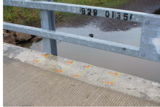
(ii) Transverse cracks over the curb
