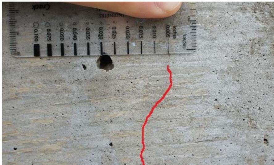
Figure 5-5. Deck slab crack width (the crack located in between beam 5 and 6 over the west abutment)
