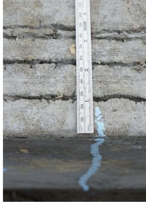
(b) Crack propagation along deck
