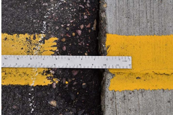
(a) Gap between the approach and bridge deck
