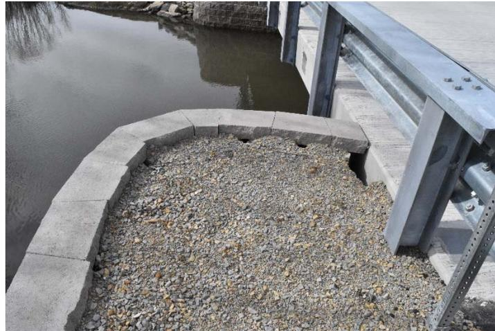
(a) Erosion of backfill material near the fascia beam
