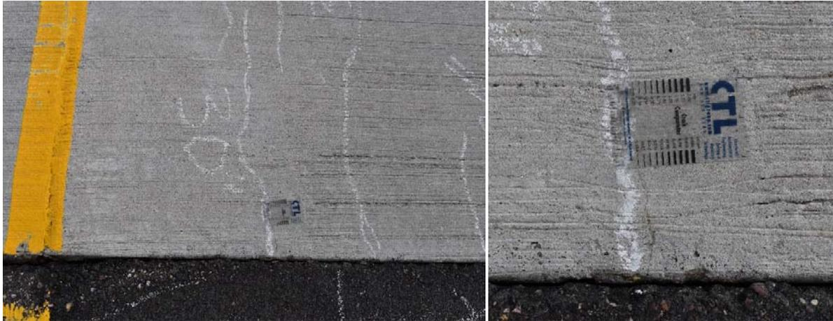
(a) Cracks over the west abutment
