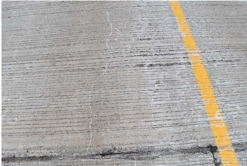
(a) Crack along the 4<sup>th</sup> shear key on east abutment
