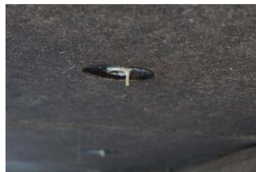
(b) Drains with moisture and efflorescence
