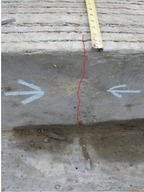
(a) Full-depth deck slab crack
