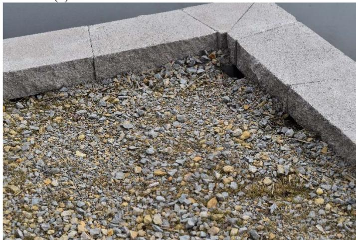
(c) Erosion of backfill material at other locations
