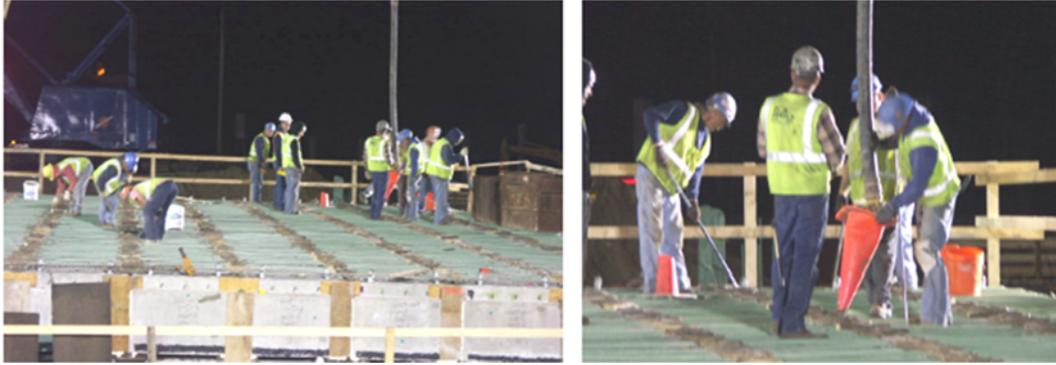
**Figure 2-11. Grouting adjacent box-beam shear keys using type R-2 grout (Oakland Drive over I-94, MI)**
