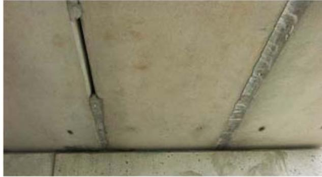
**Figure 2-3. A shear key with missing grout**
