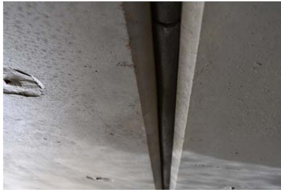
**Figure 5-13. Self-adhesive compressible sealer at the shear key**
