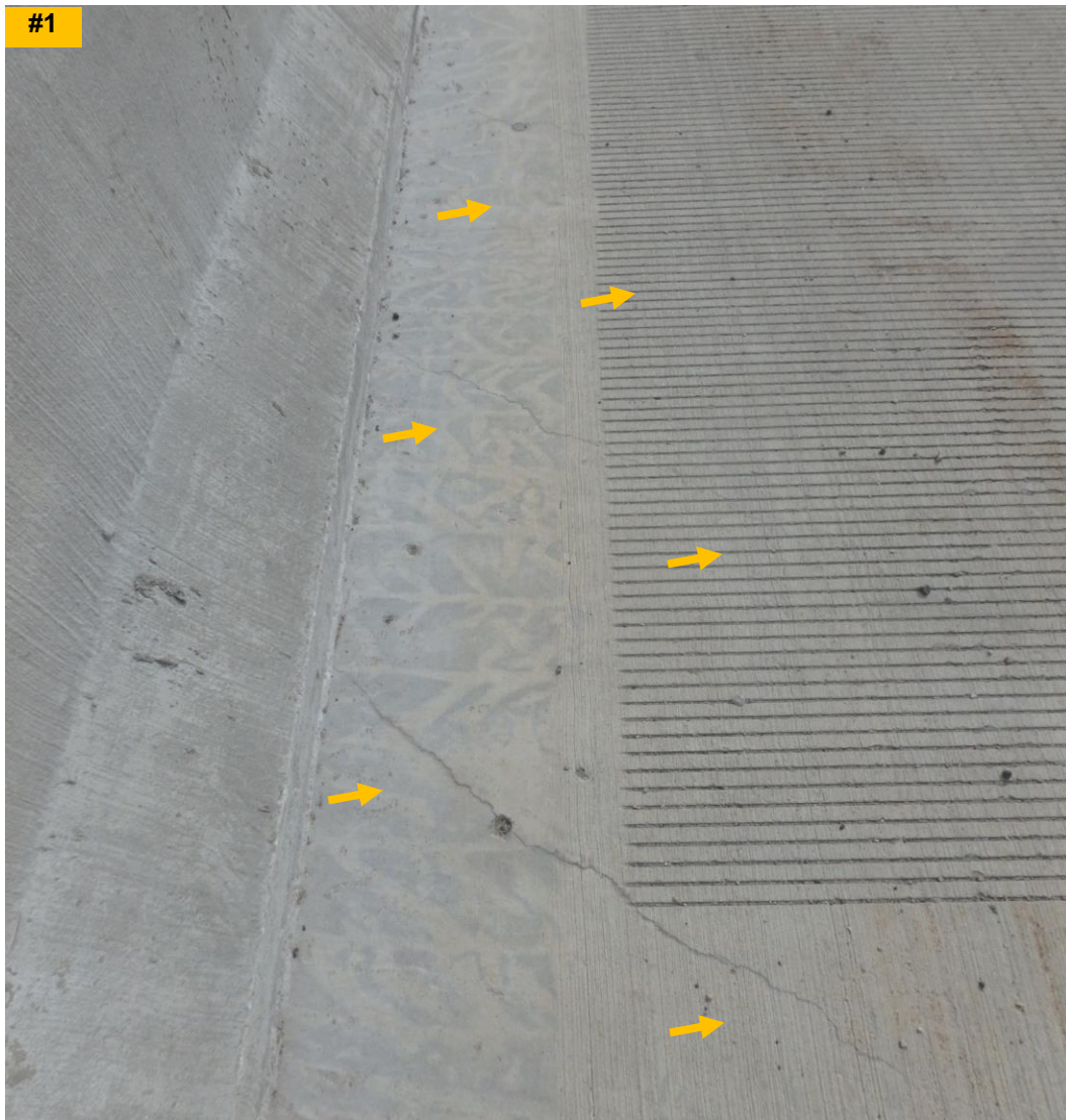
Figure A-14: IL 390 over Salt Creek – Observed Cracking Pattern (Not to Scale)
