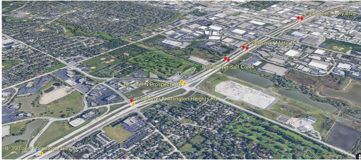
Figure A-7: An Overview of the Utilized Concrete Mixtures: Red – 90PCC1327; Yellow – 90PCC1674; Blue – 90PCC1612 (Image Obtained from Google Earth)
