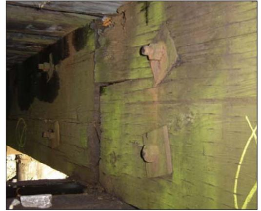
The most serious problems facing WisDOT’s timber rail bridges concern piling, including pile settlement. Note the daylight showing between the pile and cap of the timber bridge at left (page 16 of the final report). In addition, beams on the timber bridges evaluated in this study frequently showed decay at the pier caps, as seen at right (page 8 of the final report).
