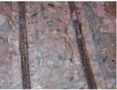
Figure 110: Close-up of TSZ(1) exposed rebar
