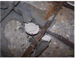
**Figure 306:** Close-up of EA-A w/A-C(1) exposed rebar after 6-months
