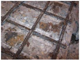
Figure 222: Close-up of Control(1) exposed rebar
