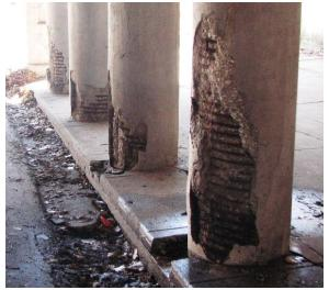
Figure 5: Spalling of concrete
