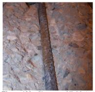
Figure 190: Close-up of T-SS(1) exposed rebar
