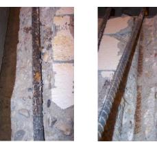
Figure 214: Close-up of EP-C exposed rebar
