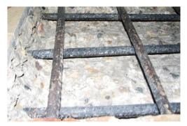
**Figure 278:** Close-up of TSZ(2) exposed rebar after 3-months
