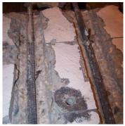
**Figure 126:** Close-up of TSZ w/EP-C(1) exposed rebar
