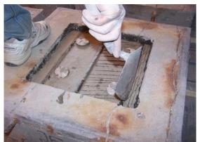
**Figure 70:** Scoring of the conventional patch repair material after the first lift had reached final set
