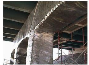
Figure 24: Operational ECE system <sup>(91)</sup>
