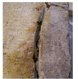
**Figure 63:** Presence of cracking exposed through routing
