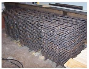
Figure 43: Layers of prepared reinforcement
