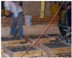
**Figure 49:** Placing the bottom layer of concrete with mixed-in chlorides
