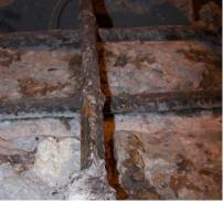
Figure 182: Close-up of EA-B(2) exposed rebar
