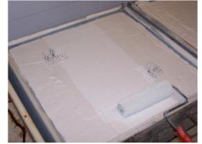
**Figure 38:** Application of polyurethane coating to epoxy coating
