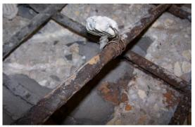
**Figure 298:** Close-up of EA-A(2) exposed rebar after 6-months
