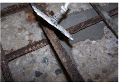
**Figure 258:** Close-up of TSZ w/EP-C(1) exposed rebar after 6-months
