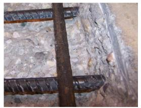
Figure 62: Loss of ribs on reinforcing steel
