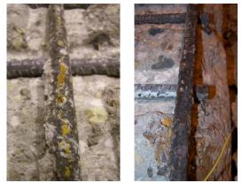
Figure 230: Close-up of Control(2) exposed rebar
