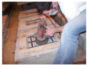
**Figure 61:** Cleaning of the reinforcing steel by wire brush
