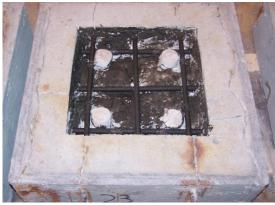
**Figure 68:** Application of bonding agent to substrate (not applied on or directly below anodes)
