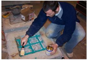
Figure 71: Applying the concrete primer for EM
