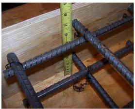
Figure 44: Clear cover to reinforcement
