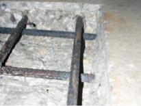
**Figure 270:** Close-up of TSZ(1) exposed rebar after 3-months
