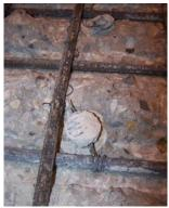
**Figure 142:** Close-up of EA-A w/A-C(1) exposed rebar
