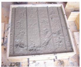
**Figure 50:** Placement of the middle layer of concrete with mixed-in chlorides
