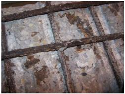
**Figure 174:** Close-up of EA-B(1) exposed rebar
