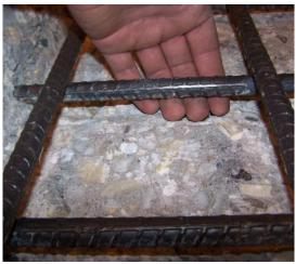
Figure 60: "Finger-gap" below reinforcing steel
