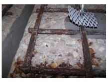
**Figure 274:** Close-up of TSZ(1) exposed rebar after 6-months
