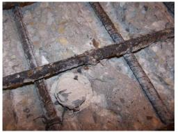
Figure 166: Close-up of EA-A(2) exposed rebar
