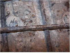
Figure 158: Close-up of EA-A(1) exposed rebar
