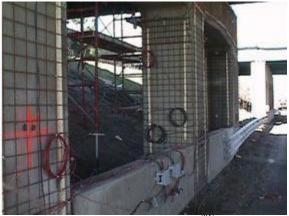
Figure 22: Installation of steel mesh <sup>(91)</sup>
