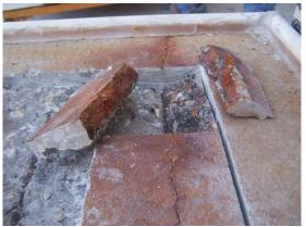
Figure 58: Discoloration of concrete discovered during concrete removal
