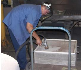
Figure 33: Grit blasting of the concrete surface
