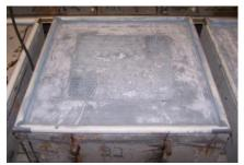
**Figure 279:** Condition of TSZ(2) after patch repairs
