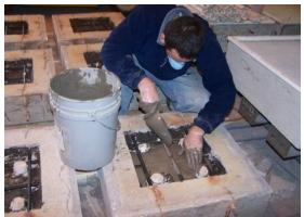
**Figure 69:** Placing the conventional patch repair material
