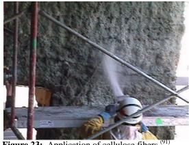
Figure 23: Application of cellulose fibers <sup>(9</sup>
