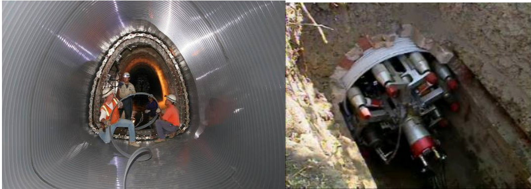
Figure 3-7 Manual Installation (ASCE, 2008).
