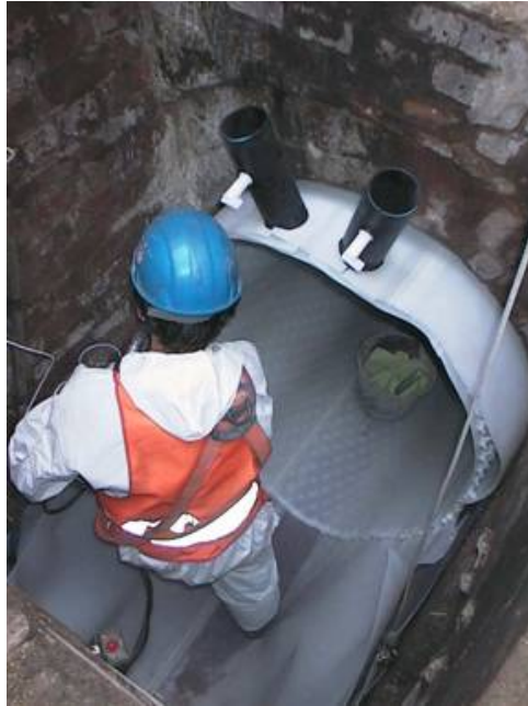
Figure 3-23 Attachment of grouting ports (ASCE, 2008).
