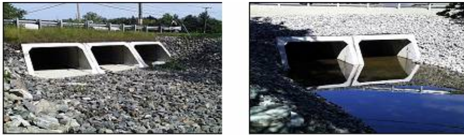
Figure 1-9 Multiple Barrel Culverts (Source: American Concrete Industries, 2008)
