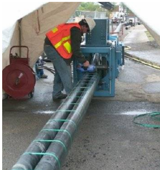
Figure 3-10 Mechanically folded liners equipment and pipe. (Source: Insituform Technologies)
