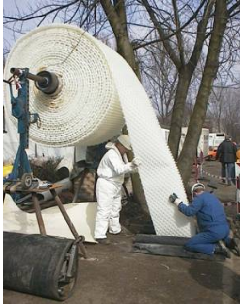
Figure 3-21 Insertion of the anchored liner (ASCE, 2008).
