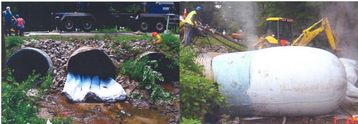
Figure 3-3 Pull and Inflate process (NASSCO, 2007).
