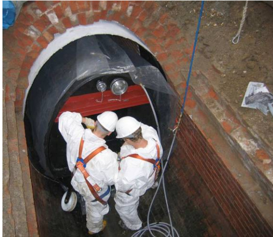
Figure 3-24 Plugging of the HDPE FIPP ends (ASCE, 2008).
