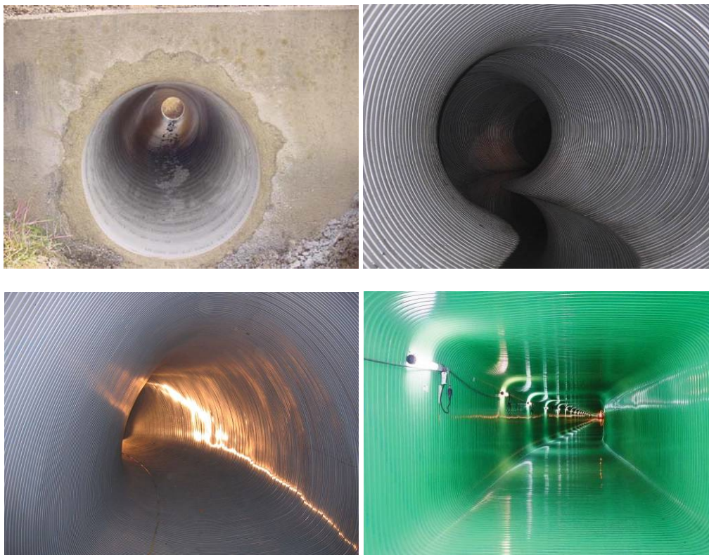
Figure 3-5 Different rehabilitated culvert shapes (ASCE, 2008).
