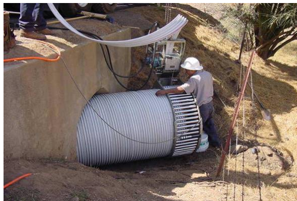
Figure 3-6 Spiral wound stationary winding machine (ASCE, 2008).
