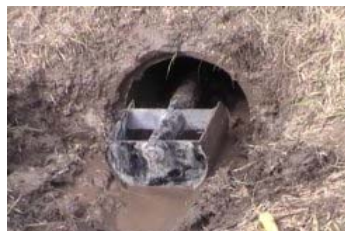
Figure 4-3 Pull Bucket (ASCE, 2008)
