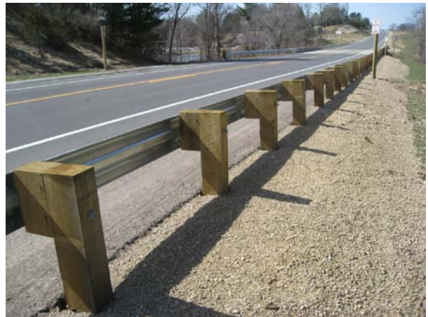
Figure 21 – View of the new guardrail post installations at Royalton site (left) and Merrimac site (right).
