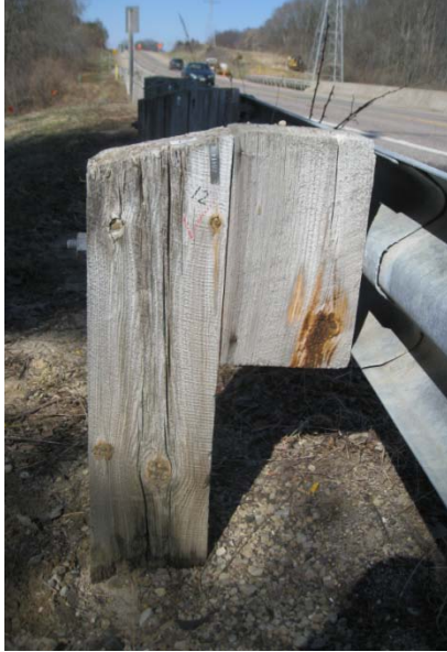
Figure 7 – Condition of old guardrail posts after several years of service near Merrimac, Wisconsin.
