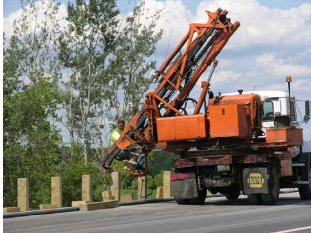
Figure 20 – Installation of new guardrail posts at the field test sites using a pneumatic machine.
