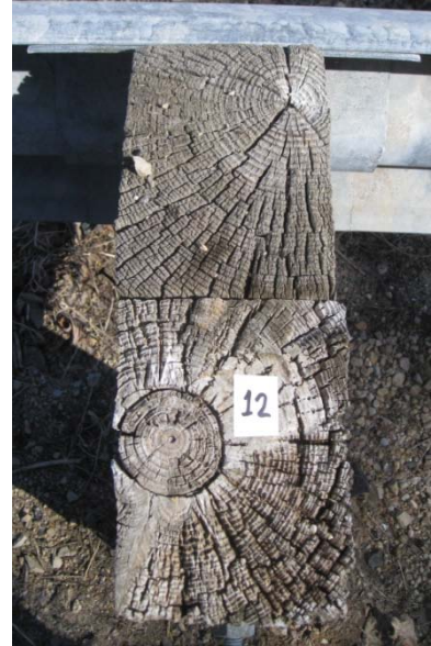
Figure 7 – Condition of old guardrail posts after several years of service near Merrimac, Wisconsin.
