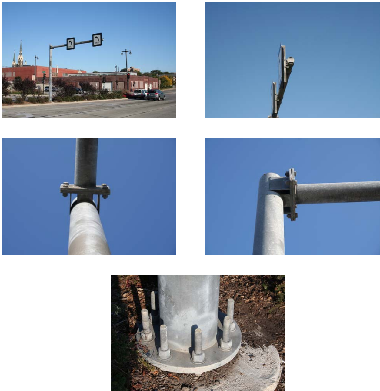
Figure 2.7 Monotube Cantilever Sign Support Structure Over Sixth Street in Milwaukee, Wisconsin.
