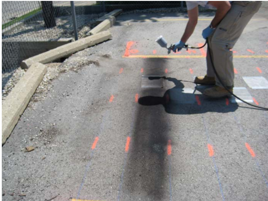
Figure 4.4. Spray Gun Application of CSS-1h
