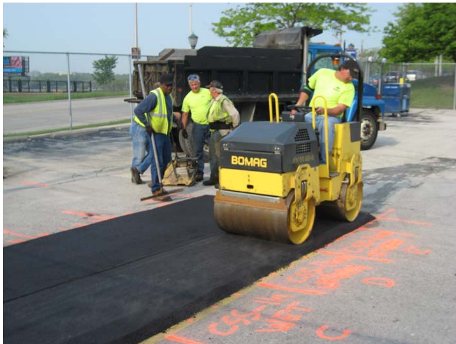
Figure 4.11. Final Compaction With Steel Wheel Roller
