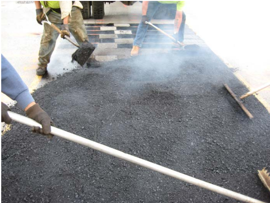
Figure 4.9. Spread of HMA Materials
