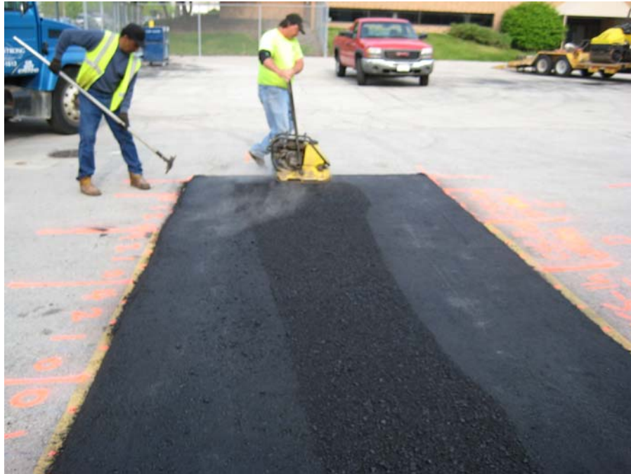
Figure 4.10. Edge Compaction with Plate Compactor
