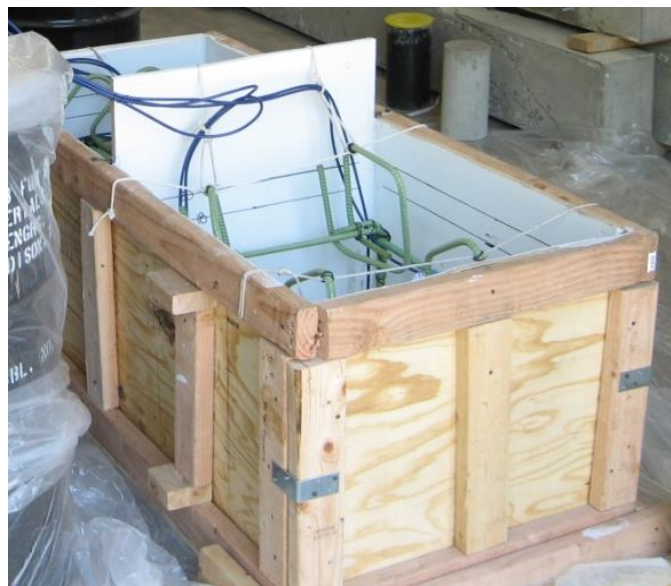
Figure 2.40 Exterior of column formwork shows supports along the length and width and connections in shear
