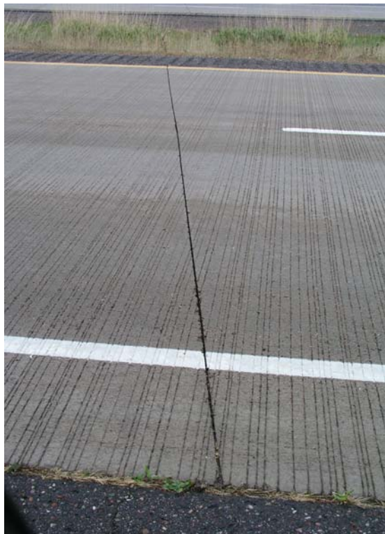
Figure 4.4.5 Typical Chipped Joint – WIS 29 Abbotsford
