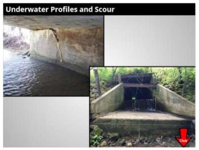
Underwater profiles are generally not needed for box and pipe culverts, as the floor is part of the structural system. Box culvert settlement due to scour or loss of fill can cause serious problems. While under water profiles are not required for Cstructures with structural floors (box culverts), the flow lines, inlets and outlets should be probed for irregularities during inspections and after major flood events to determine if undermining and scour are present.
