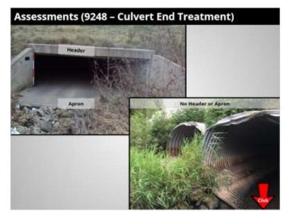
The assessment Culvert End Treatment applies to headwalls and aprons. If a culvert protrudes from the embankment without these, then this assessment would not apply (for example: steel pipe with no apron or headwall). Otherwise this assessment is to be coded as 1 for each end of the culvert.
