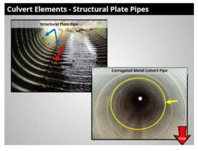
Structural plate culverts could be either steel or aluminum circular or arch culverts. They are field assembled, built-up of several precurved corrugated plates. The field assembled plate sections are fastened together with bolts to form a continuous pipe. Fastened plate edges oriented along the barrel length are called seams, while plate edges transverse to the barrel are called joints (blue arrows - note for animation only).
