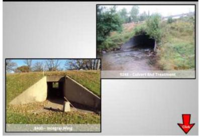
Element 8400 for integral wing walls are anchored to any combination of barrel, apron and/or headwall. Integral wings are typically reinforced concrete, but may be any material with a vertical or near vertical face. (animation - show steel culvert picture) The one exception would be steel culverts where the end of the pipe is sloped to match the embankment (see photo), although it's attached to the pipe, this is considered an end treatment.
