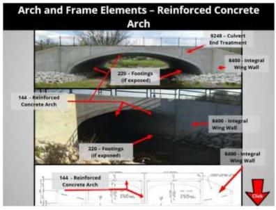
Reinforced concrete arches are the most common arch structures. These can be cast in place, but are generally precast. They can have sloped or vertical walls connecting to the main arch, but are coded the same. Elements for a reinforced concrete Arches are:
