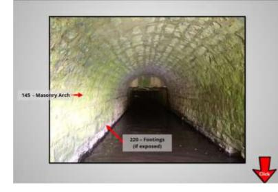
Masonry arch elements are stone or brick structures formed into the form of an arch. These structures rest on a footing, which may or may not be exposed, and have head walls and wings to retain fill.
