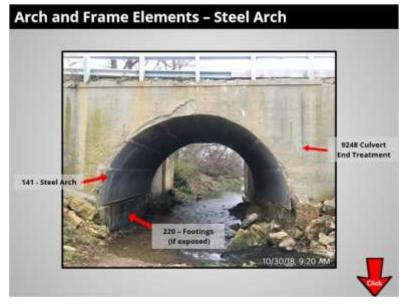
Steel arch elements are usually made up of structural plates connected to form the arch. These structures rest on a footing, which may or may not be exposed, and have head walls and wings to retain fill.
