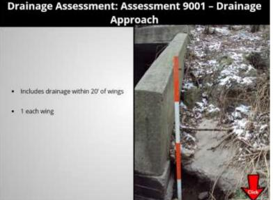
The assessment 9001 Drainage - Approach is at each quadrant of a structure and captures the condition of the drainage from the edge of roadway down the slopes behind and limited to 20 feet from the wingtip. This item is not the same as assessments 9040-9047 for the various types of slope protection, those are to be coded separately. This assessment is present on all C Structures, regardless if drainage system is present.
