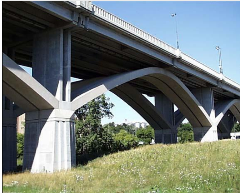
Figure 2.4.3.2-1: Open Spandrel Prestressed Arch Bridge with Struts.
