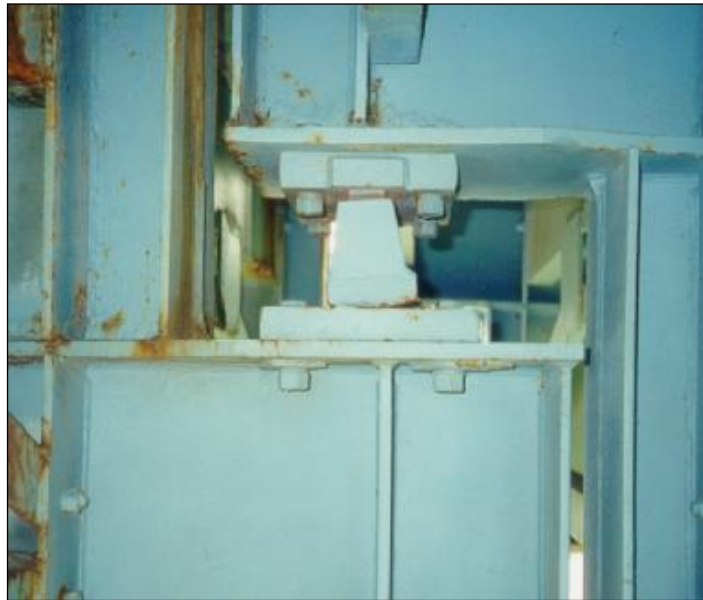
Figure 2.4.8.2-6: Rocker Bearing – Condition State 1.
