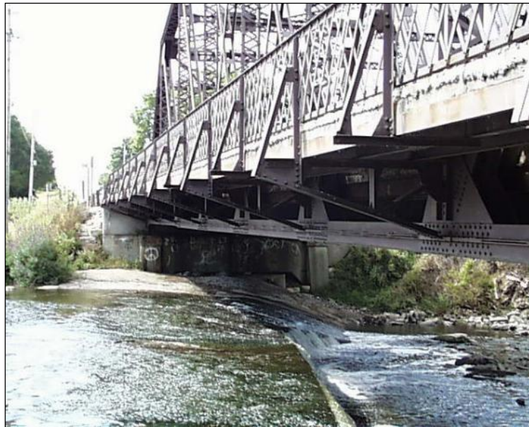
Figure 2.4.4.4-1: Truss Bottom Chord.
