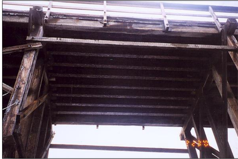
Figure 2.4.5.1-1: Multiple Timber Beams.
