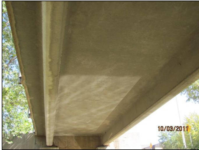
Figure 2.4.3-2: Double Tee Girder Bridge.
