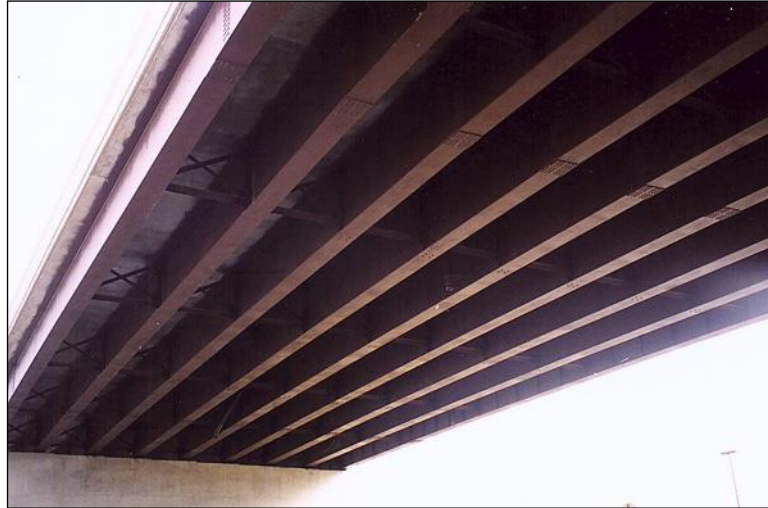
Figure 2.4.4.1-2: Fabricated Girders and Rolled Cross-Frame Members.
