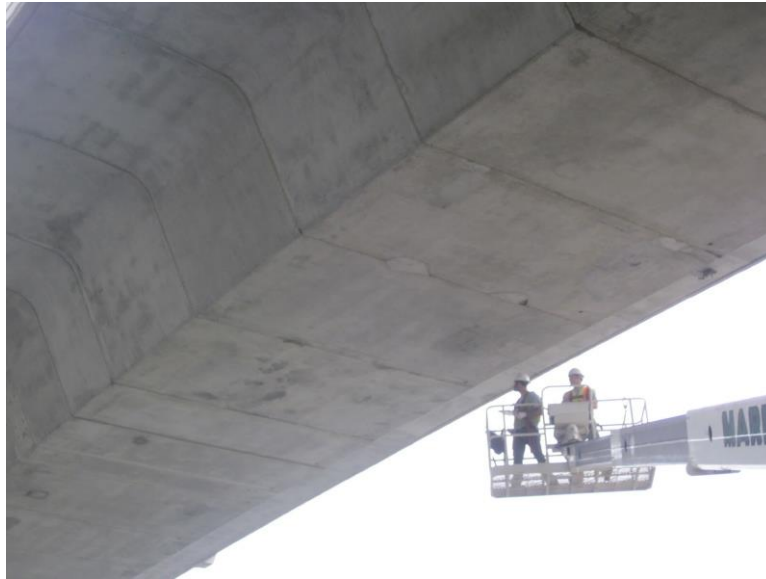
Figure 2.4.3-4: Segmental Box Girder Bridge.
