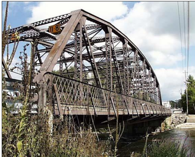
Figure 2.4.4-6: Steel Truss Bridge.
