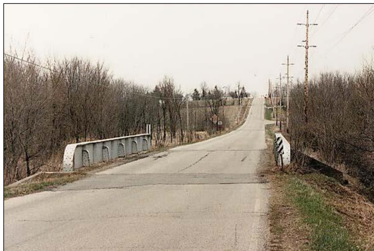
Figure 2.4.4.8-2: NSTM Through Girder Bridge.
