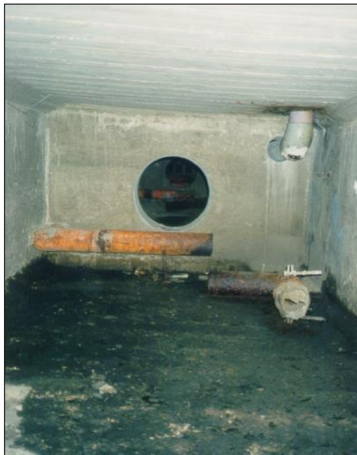
Figure 2.4.2.2-1: Inside of a Reinforced Concrete Box Girder.
