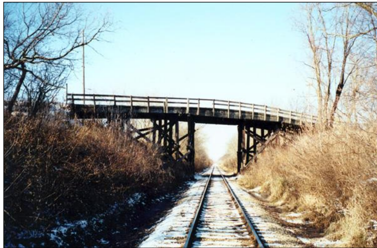
Figure 2.4.5-2: Solid Sawn Multi-Beam Bridge.
