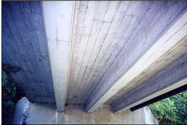
Figure 2.4.3-2: Reinforced Concrete Tee Beam Bridge.
