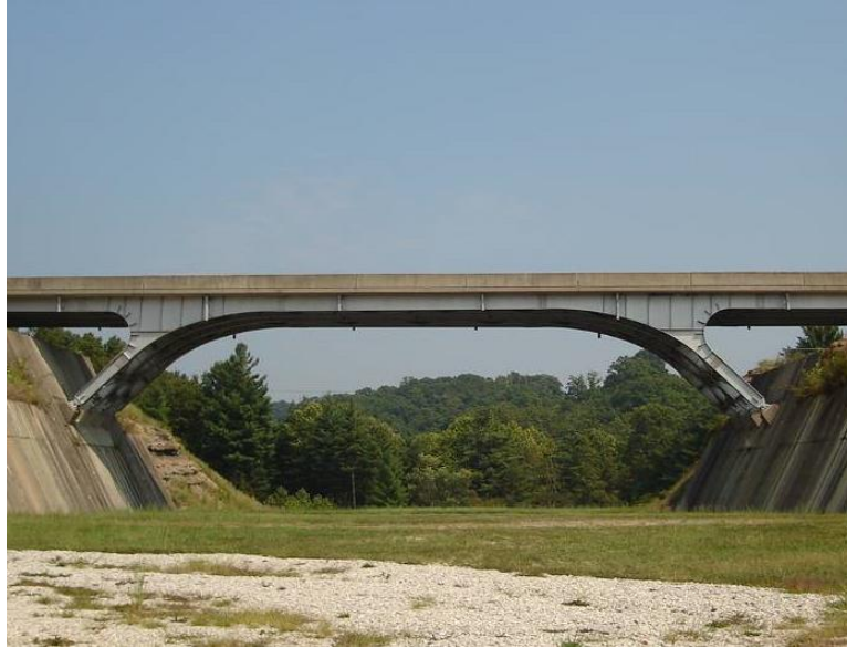
Figure 2.4.4-9: Steel Rigid Frame Bridge.
