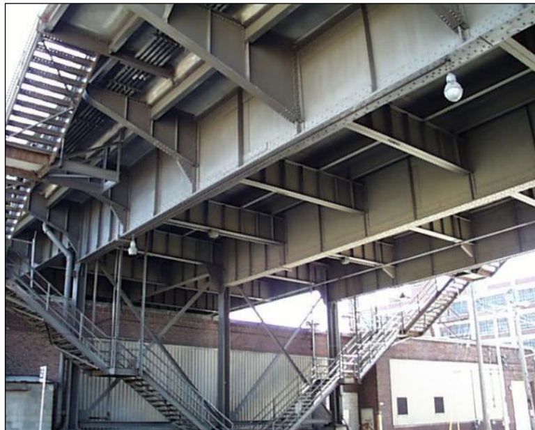
Figure 2.4.4.1-19: Fabricated Steel Girders and Floor Beams, and Rolled Stringers.
