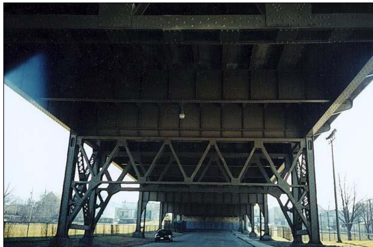
Figure 2.4.4-3: Two Girder System Bridge.
