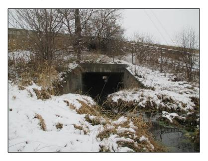
Figure 4.6.4-3: View of a single cell reinforced concrete box culvert.
