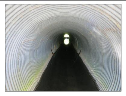
Figure 4.6.4-1: View of circular structural plate pipe culvert.
