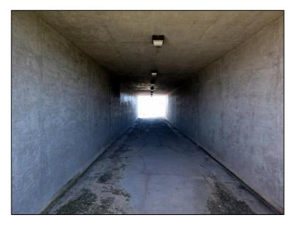
Figure 4.6.6-6: Reinforced Concrete Culvert - Condition State 1.
