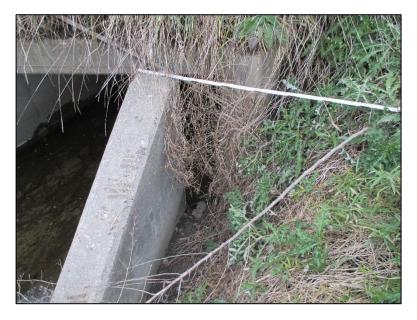
Figure 4.6.6-14: View of Wingwall Movement. Note loss of fill behind wingwall and culvert barrel – Condition State 3.
