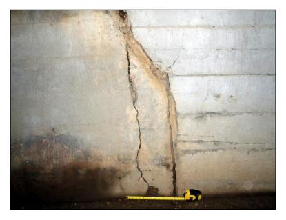
Figure 4.6.6-8: Differential Settlements Between Box Segments – Settlement Condition State 3.
