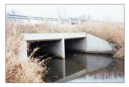
Figure 4.6.4-4: Two-cell reinforced concrete culvert.
