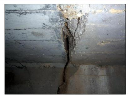
Figure 4.6.6-9: Joint Separation Between Pipe Segments – Settlement Condition State 3.
