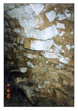
Figure 4.6.6-10: Masonry Culvert with Severe Deterioration of Mortar Joints.
