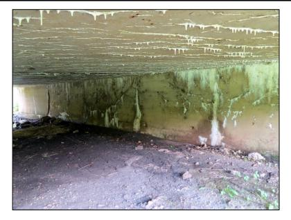
Figure 4.6.6-7: Deterioration on Culvert Wall – Heavy Density Cracking with Efflorescence Condition State 4.
