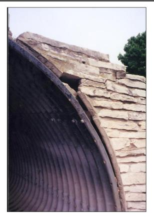
Figure 4.6.7-2: Masonry headwall separating from the barrel.
