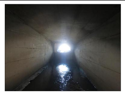
Figure 4.6.4-5: View of reinforced concrete single cell box culvert with corrugated steel pipe arch extension
