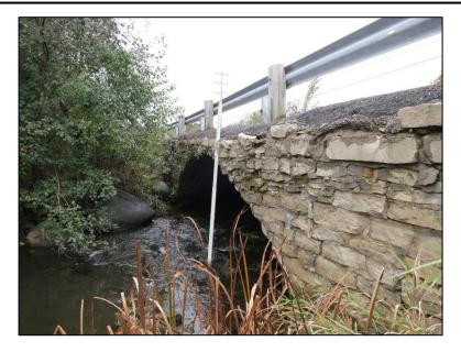
Figure 4.6.4-2: View of a corrugated steel arch culvert with masonry headwalls.
