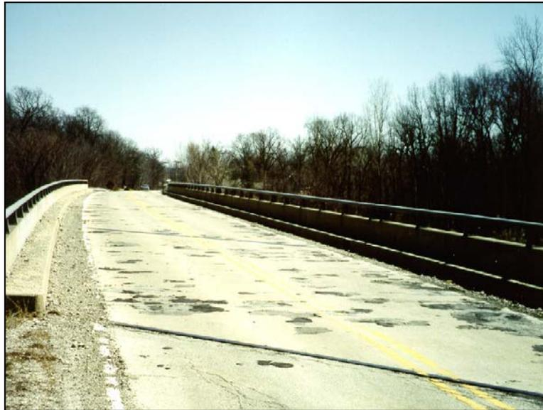
**Figure 5.11.1-1:** Bridge Deck with Asphalt Overlay and Extensive Patching.
