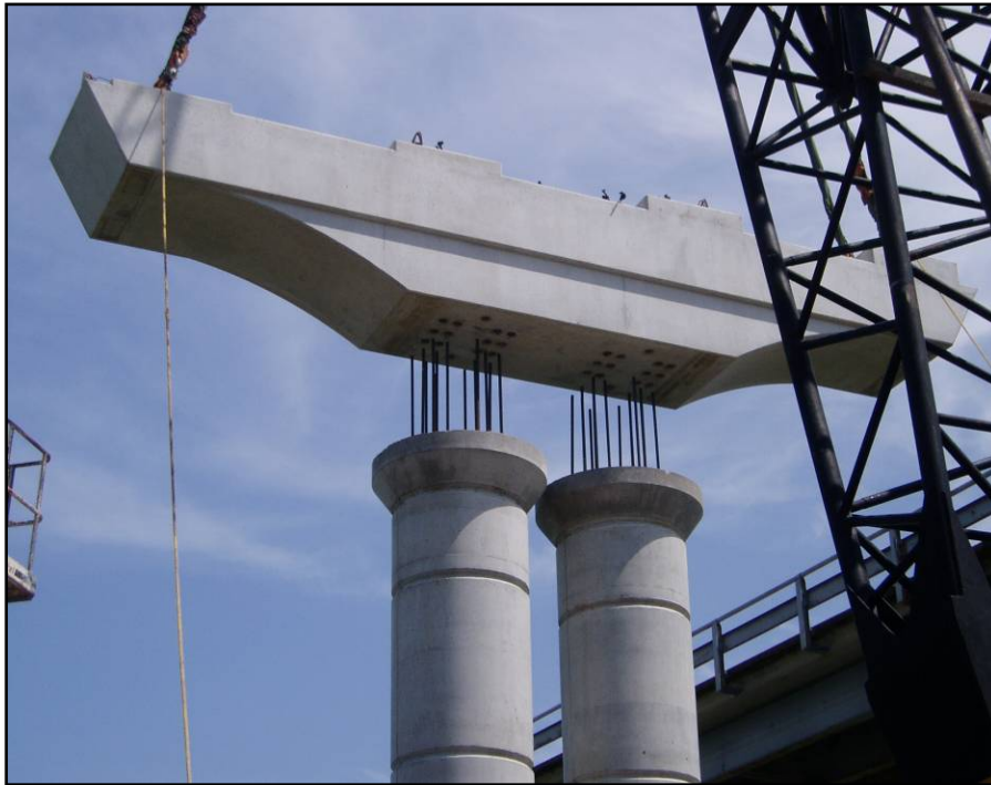
Figure 7.1-1 Prefabricated Pier Cap
