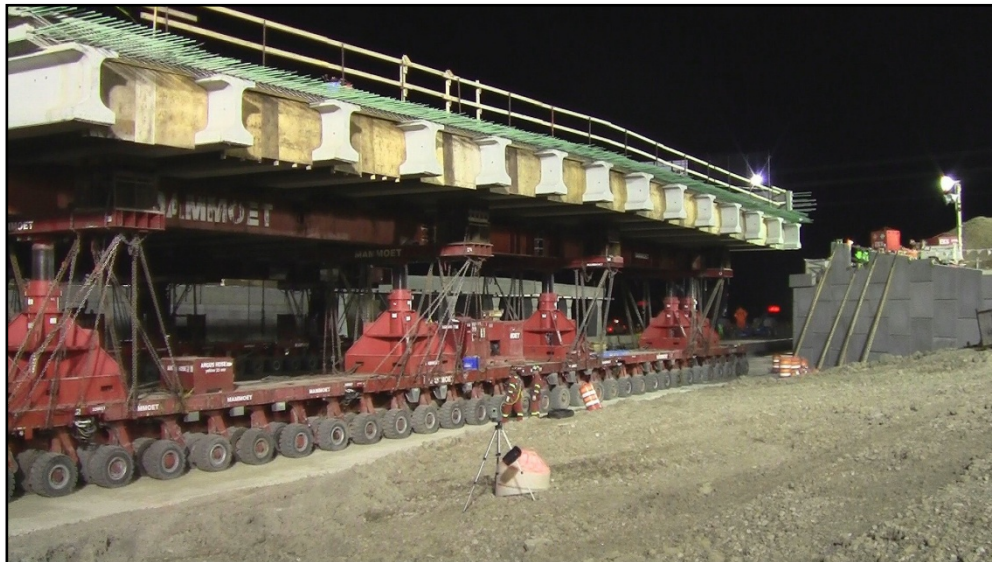
Figure 7.1-7 Self Propelled Modular Transporters Moving a Bridge
