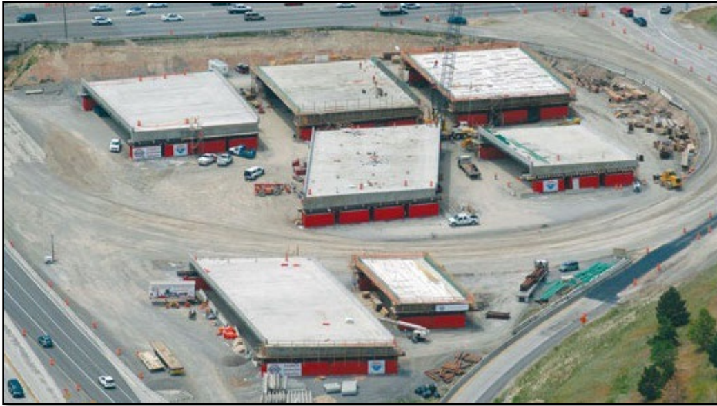
Figure 7.1-8 Example Bridge Staging Area (BSA)
