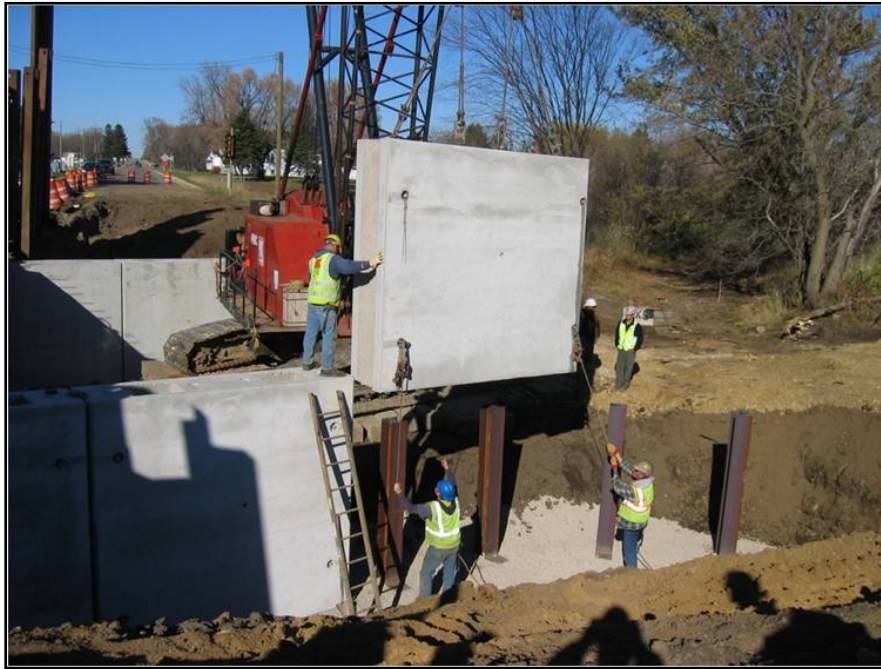
Figure 7.1-2 Prefabricated Abutment
