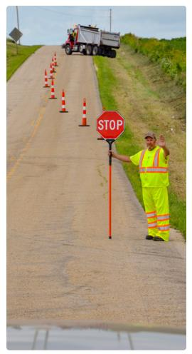
Figure 3: Stopping first vehicle from shoulder
