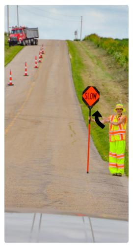
Figure 5: Releasing traffic into the open lane; standard drive lane
