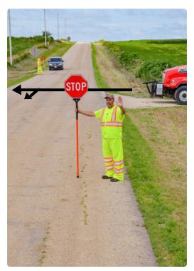
Figure 9: Stopping traffic for left-turning vehicles
