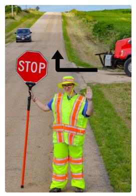
Figure 10: Stopping traffic for right-turning vehicles
