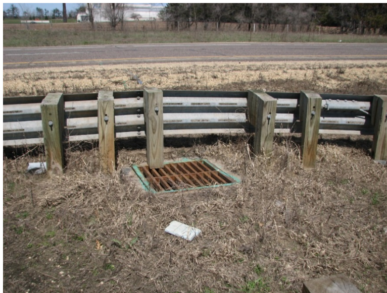
Figure 20.44 Drainage and Safety Hardware Installation Not Coordinated
