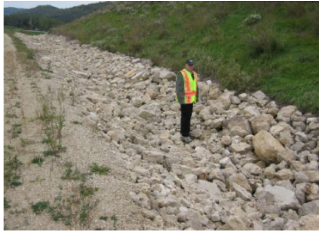
Figure 20.10 Riprap is a Hazard 13
