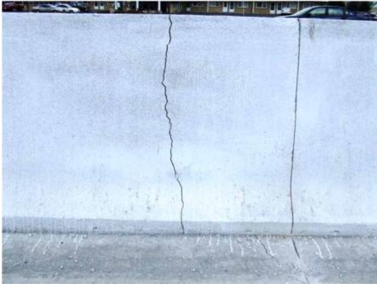
Figure 30.61 Cracked Concrete Barrier Needing Repair
