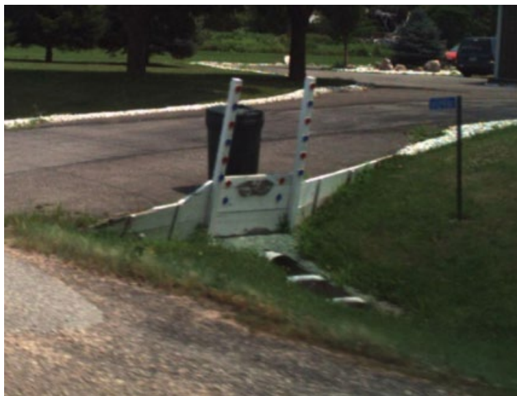
Figure 20.3 Installation of a Traversable Culvert but Retaining Wall is a Hazard
