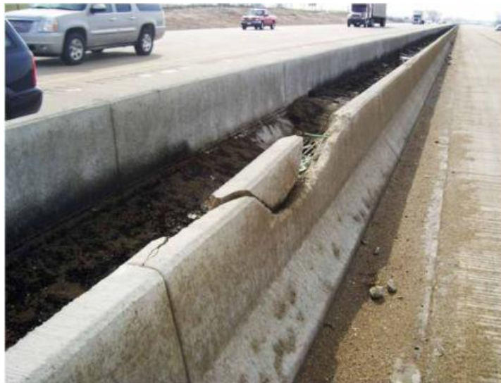
Figure 30.59 Cracked Concrete Barrier Needing Repair
