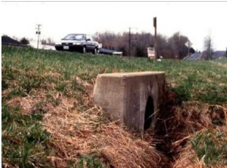
Figure 20.6 Headwall for Culvert Pipe is a Hazard xv10
