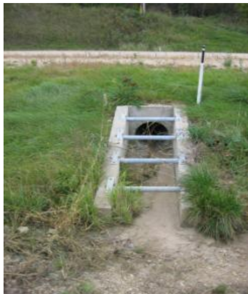
Figure 20.7 Pipes are Installed Parallel to Direction of Travel 11 Hazard
