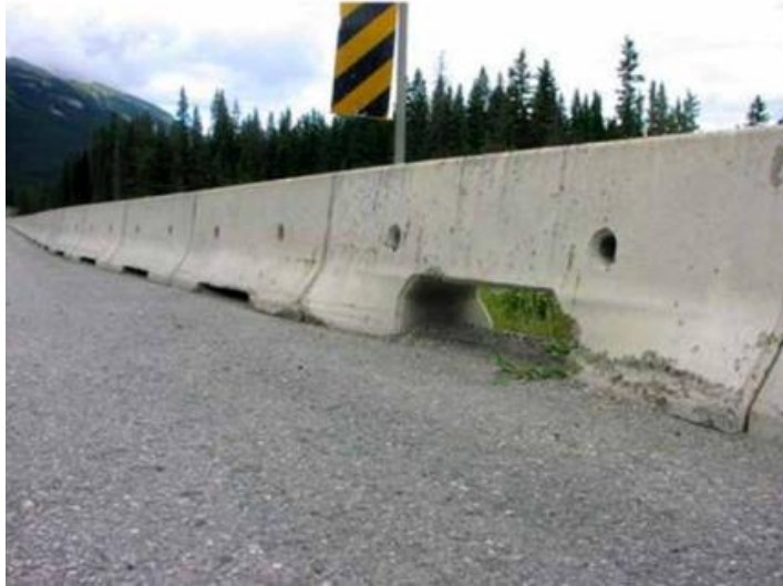
Figure 30.58 Opening in barrier that can snag a vehicle cvi
