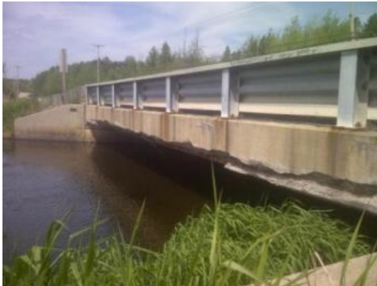
Figure 20.15 Damage to Side of a Deck that May Influence Parapet Performance
