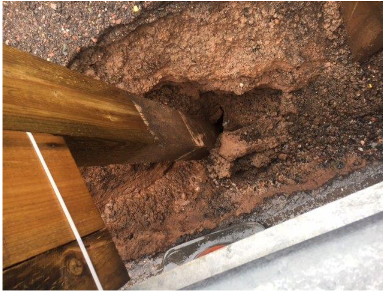
Figure 30.12 Post Driven Into a Culvert
