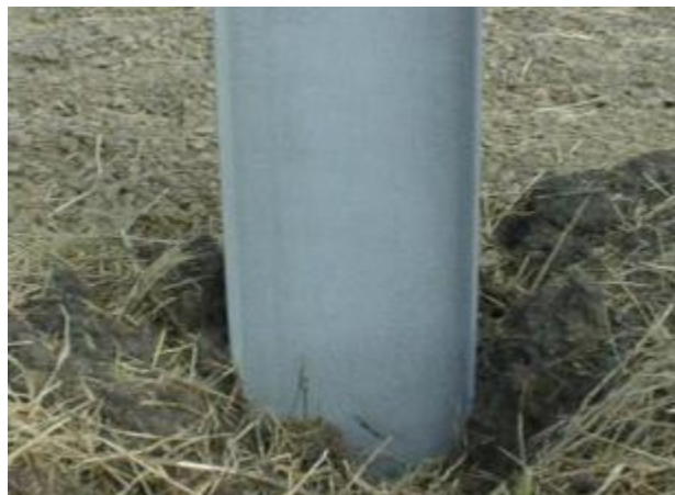
Figure 20.22 Buried Breakaway Feature xxix
