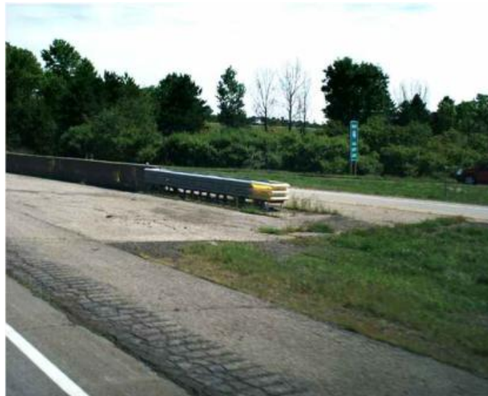
Figure 30.73 Photo of GREAT installation
