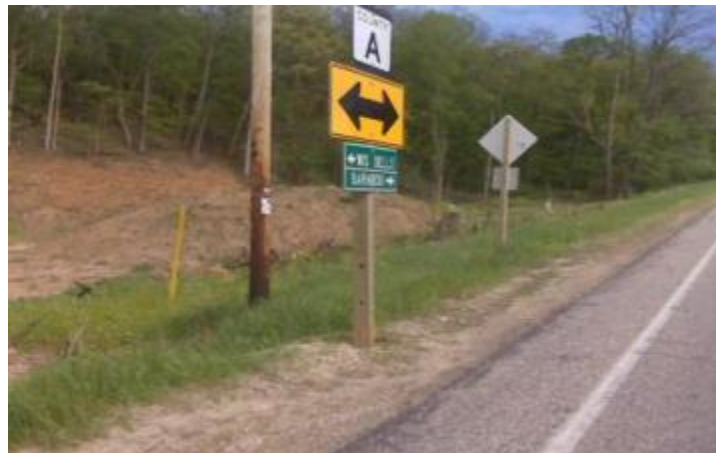
Figure 20.23 Breakaway Holes are too High 22
