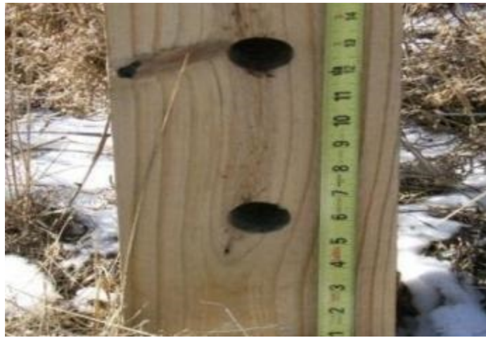
Figure 20.24 Breakaway Holes in the Wrong Location xxx
