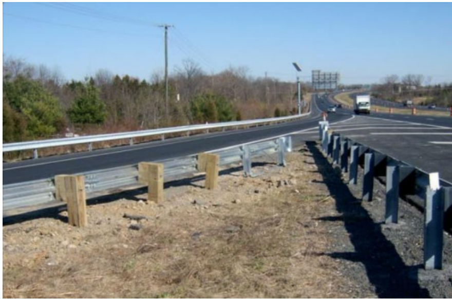
Figure 30.30 End Treatment Placed Near Each Other lxxix
