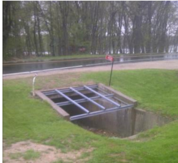
Figure 20.9 Grate Should Have Covered All of the Opening 12 Hazard
