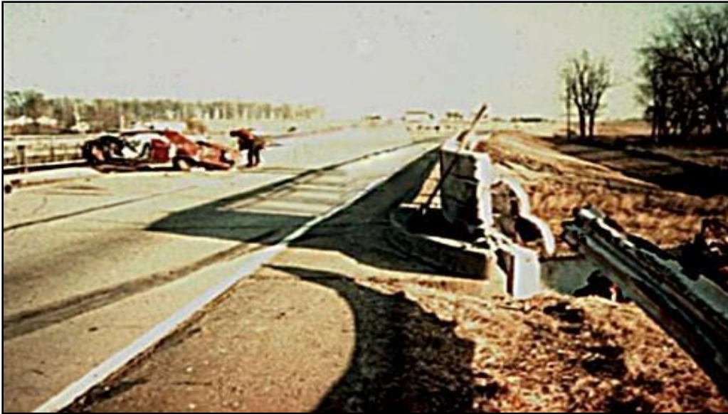
Figure 30.48 Unconnected Beam Guard Gated or Directed Vehicle into Blunt End ci
