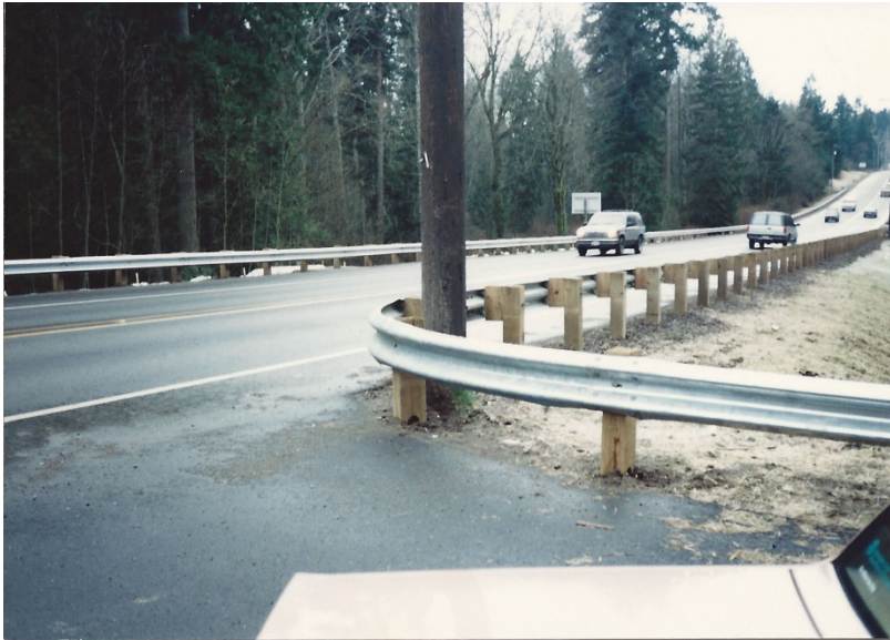
Figure 30.14 Utility Pole Will Prevent Proper Operation of Short Radius System lxvii
