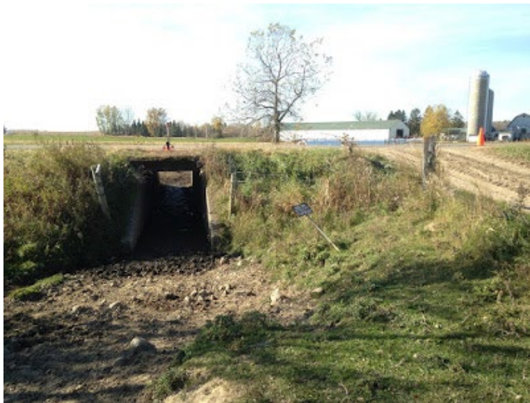
Figure 30.80 Culvert by Driveway
