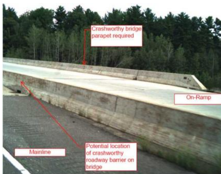
Figure 30.25 Crashworthy Barrier on Bridge
