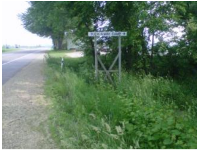
Figure 20.21 Non-Breakaway Sign
