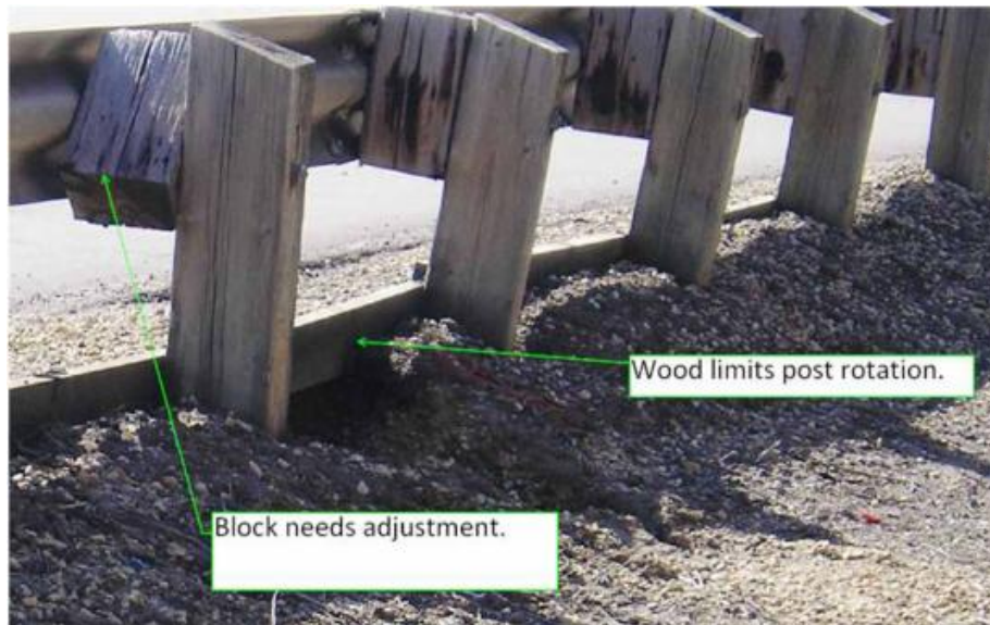
Figure 30.40 Wood planks limit post rotation
