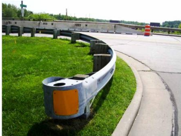
Figure 30.54 Problematic Short Radius with installation Problems
