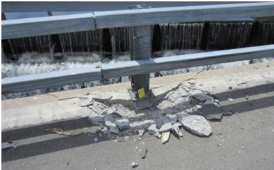
Figure 20.16 Strength of Barrier Connection Critical to Barrier Performance and Structural Maintenance
