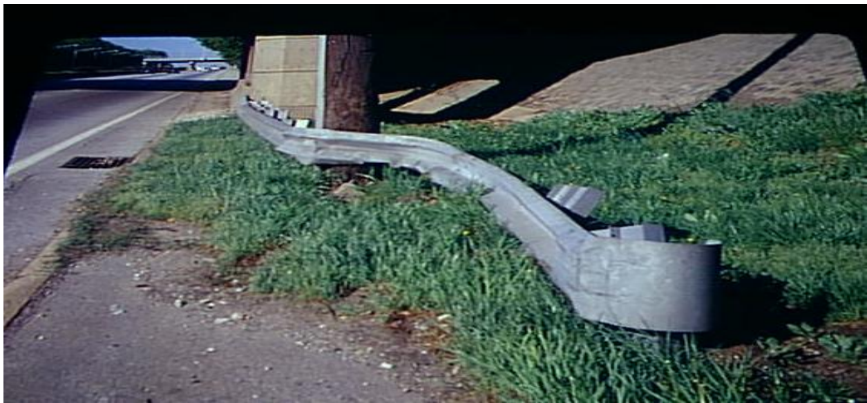
Figure 30.39 Beam Guard Directed Vehicle into Utility Pole xcviii, 53
