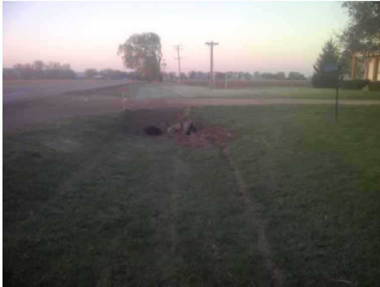
Figure 20.4 Vehicle Hit a Hazardous Driveway Slope
