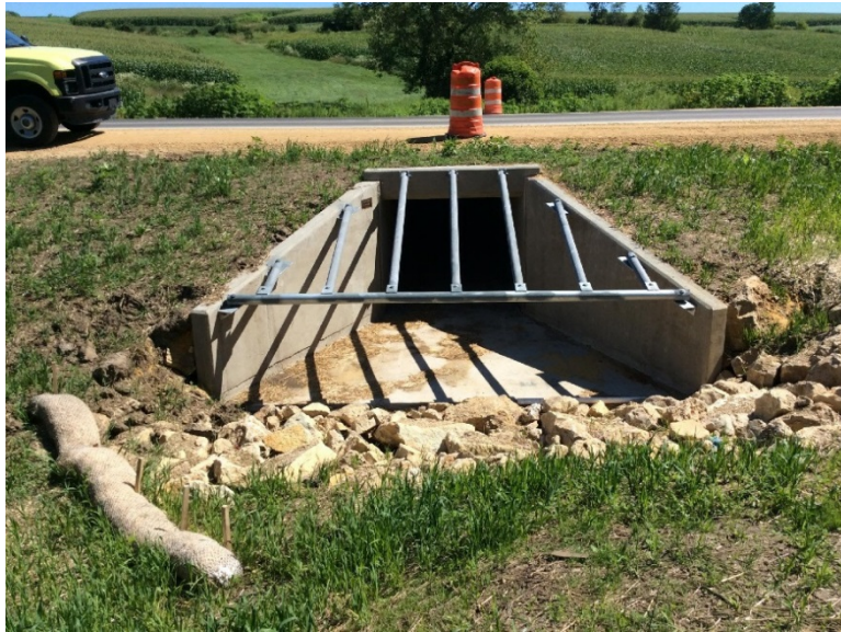
Figure 20.8 Grate Does Not Extend to Bottom of Apron End Wall or Culvert xvi Hazard
