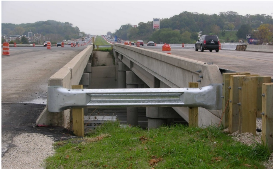
Figure 15.13 Beam Guard Installed in Median Gap Between Bridges
