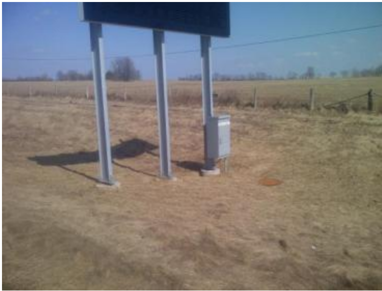
Figure 20.30 Message Board is too Heavy for Breakaway Features 24
