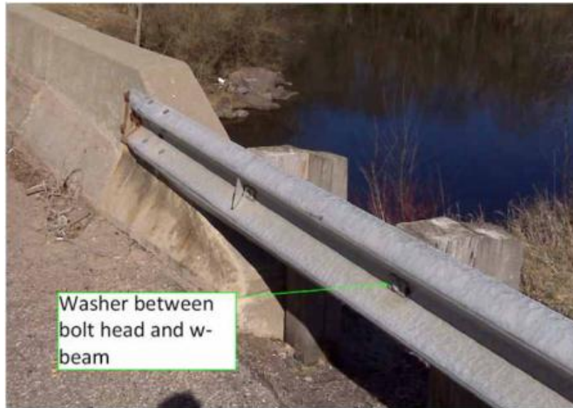
Figure 30.42 Beam Guard Transition to Rigid Barrier
