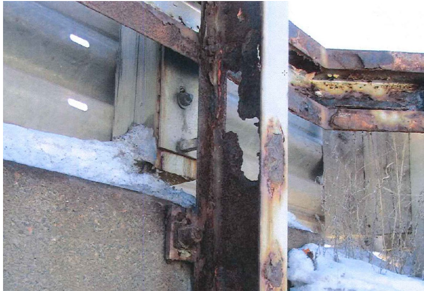
Figure 20.14 Roadway Project Significant Damage to Bridge Railing
