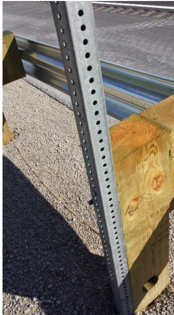
Figure 30.36 Sign Mounted on Beam Guard
