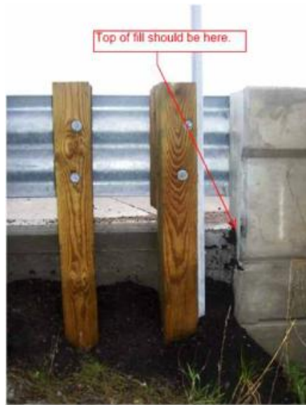
Figure 30.44 Problematic Thrie Beam Transition to Rigid Barrier
