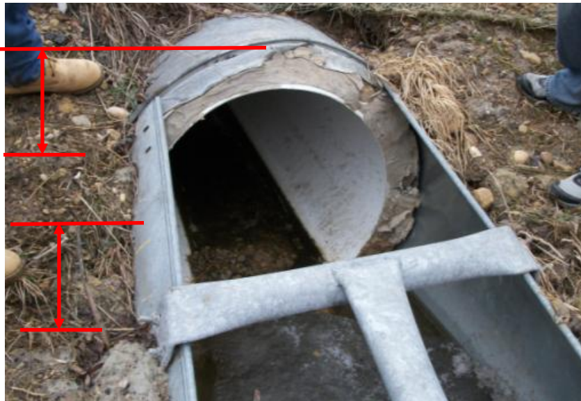
Figure 20.34 Portions of Endwall and Culvert are 4-inch Hazard on 5-foot Chord
