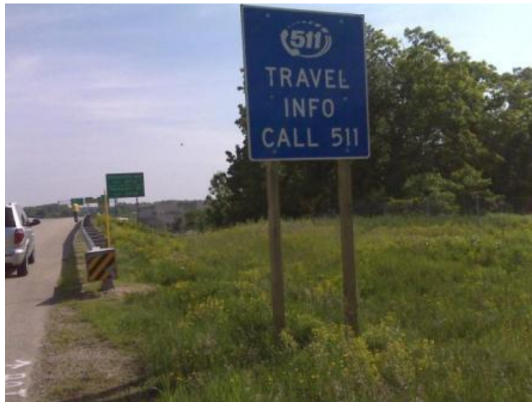
Figure 30.29 Fixed Object may Funnel Vehicle into EAT
