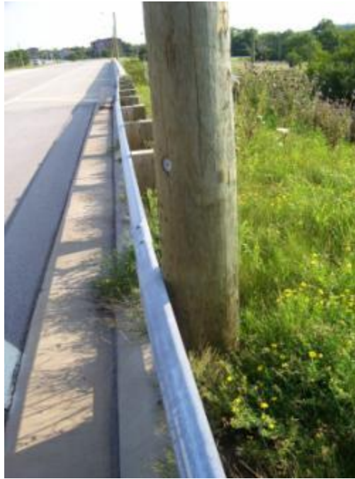
Figure 30.38 Utility Pole placed within Working Width of Barrier
