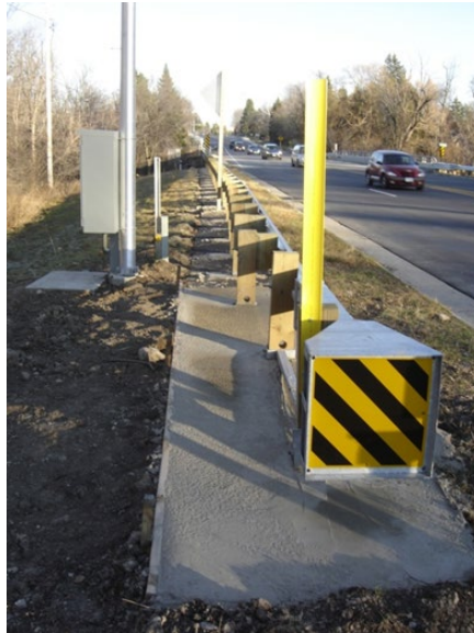
Figure 20.45 ITS and Safety Hardware Installation Not Coordinated
