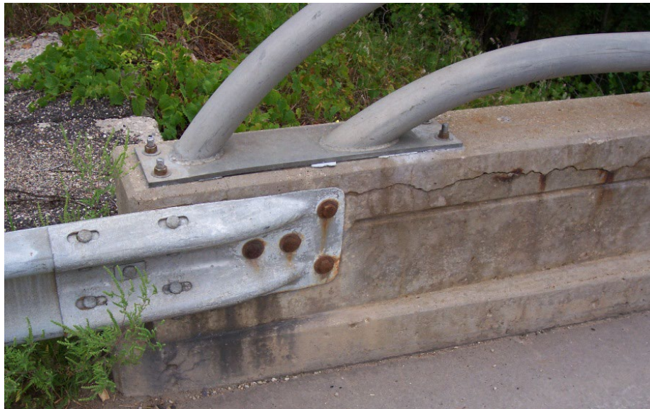
Figure 30.47 Damage to Parapet and Height of Parapet Issues
