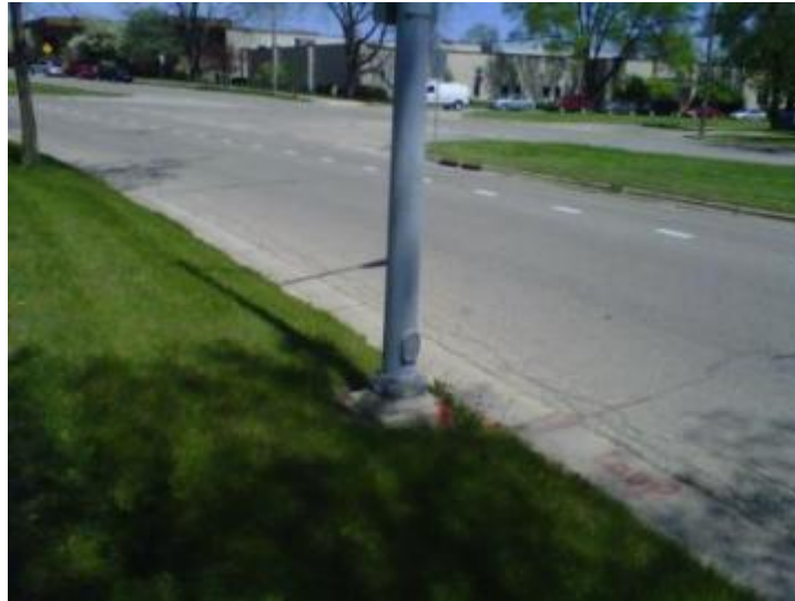
Figure 20.19 Light Pole using Non-Breakaway Hardware 20
