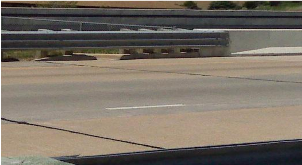
Figure 30.43 Thrie Beam Missing Posts
