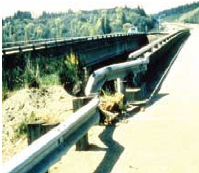
Figure 30.49 Pocket Formed by Vehicle Hitting Beam Guard Connected to Parapet cii
