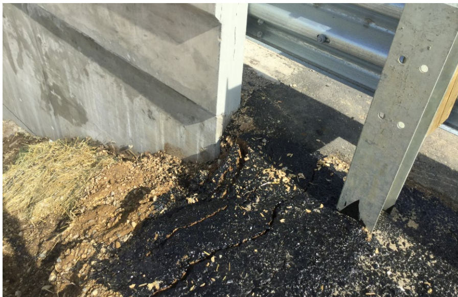
Figure 30.45 New Thrie Beam Transition with Drainage Problems
