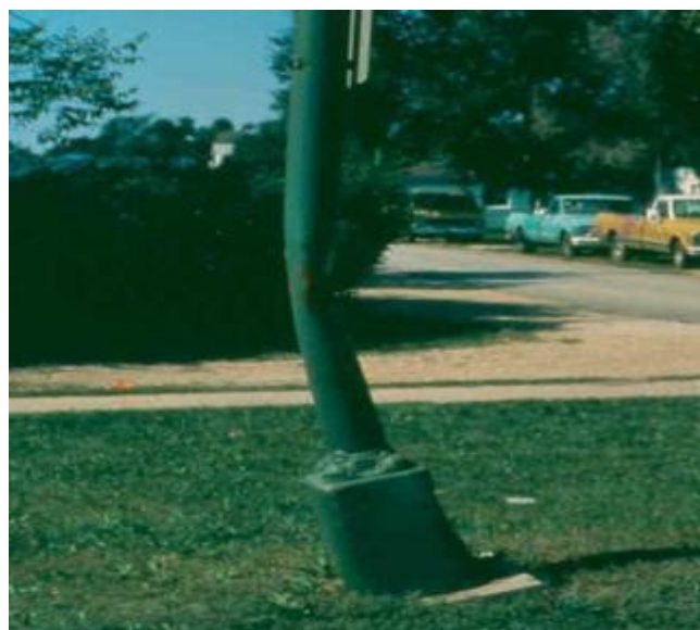
Figure 20.29 Grading Leads to Improper Pole Engagement xxxiv
