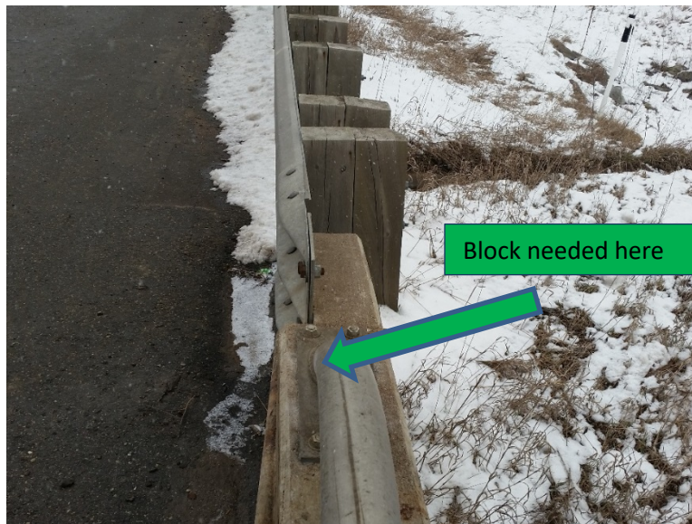
Figure 30.46 Missing Wood Block is a Snag Point
