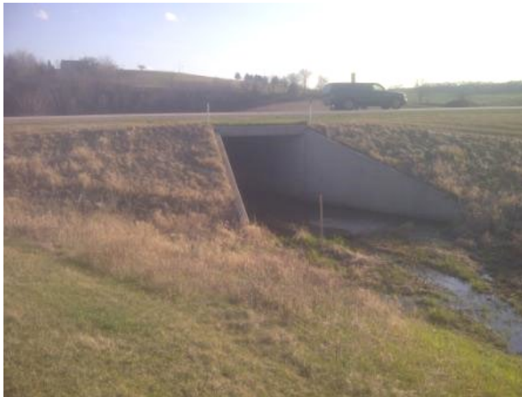
Figure 30.78 Overall height of this box culvert would need shielding. Edge of box culvert is just beyond clear zone.
