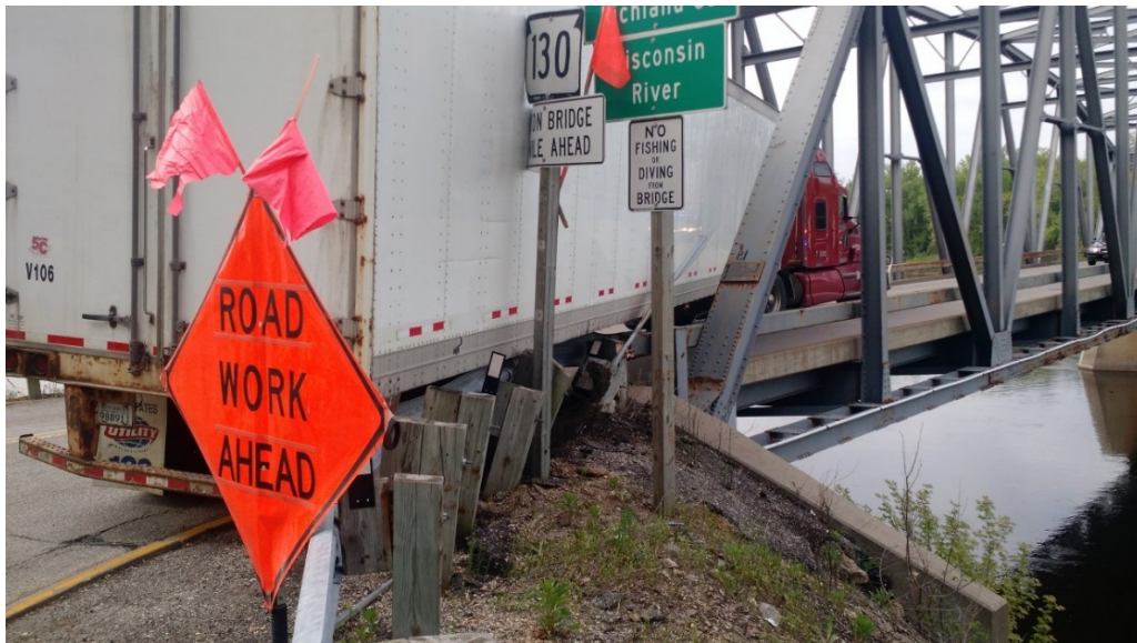
Figure 30.13 Truck Hung Up on Thrie Beam Transition and Short Radius
