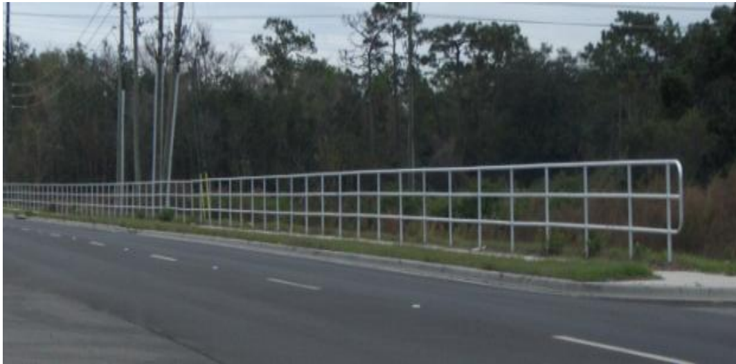
Figure 20.17 The Pedestrian Rail is a Hazard xxvii
