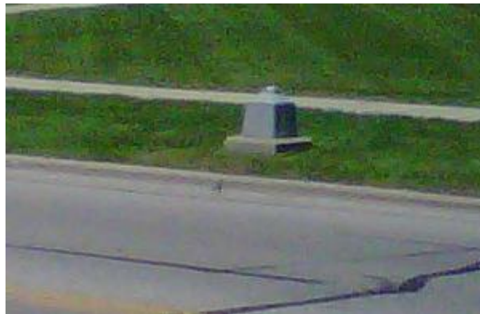
Figure 20.20 The Footing is a 4-inch Hazard 21
