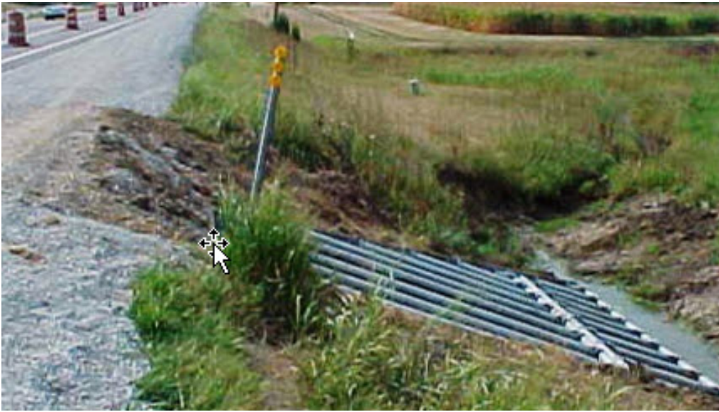
Figure 30.79 Larger Traversable Grate 62
