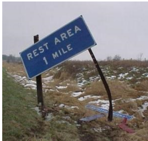
Figure 20.25 Cor-Ten/Weathering Steel Prevented Breakaway Hardware from Working xxxi 23
