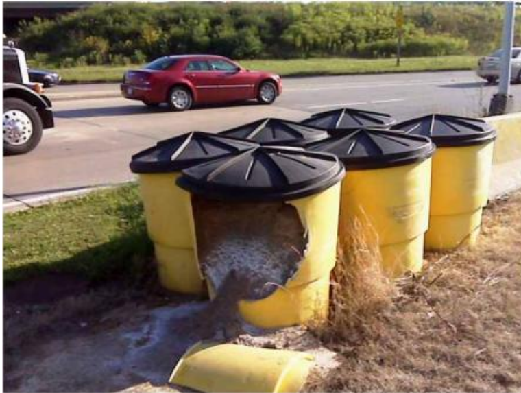
Figure 30.74 Problematic Sand Barrel Array
