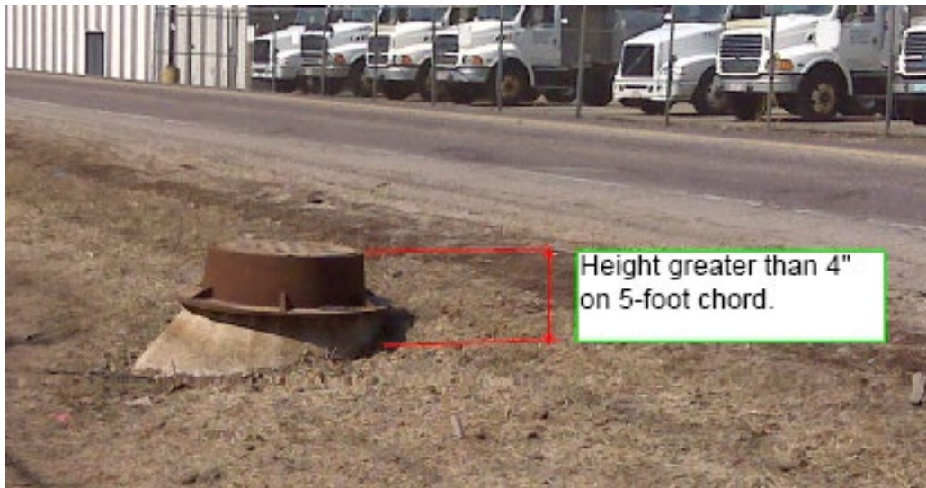
Figure 20.33 Manhole is Fixed Object Hazard
