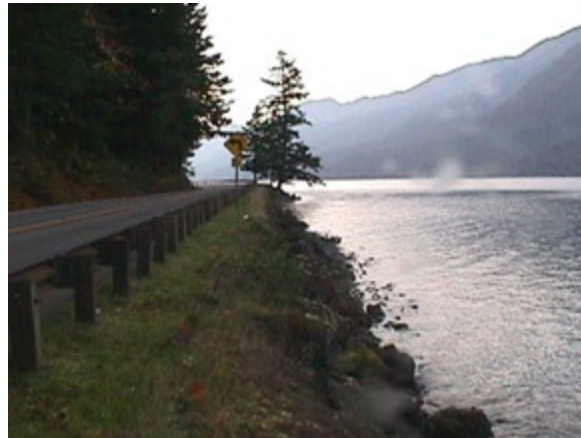
Figure 20.11 Shielding Hazardous Water
