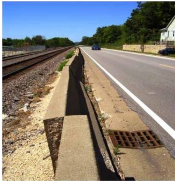
Figure 30.56 Concrete Barrier Tipping Over
