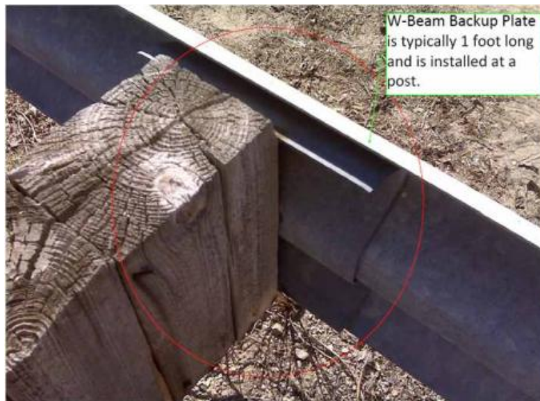
Figure 30.37 W-Beam Backup Plate
