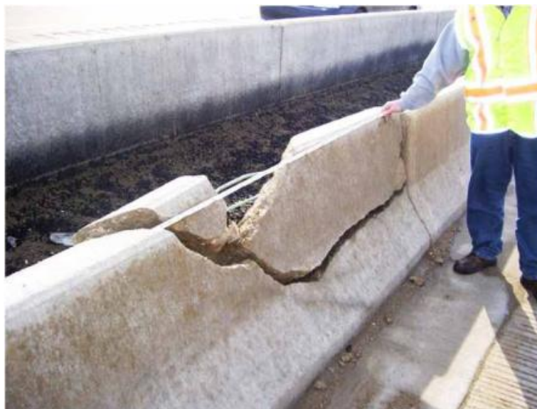
Figure 30.60 Cracked Concrete Barrier Needing Repair
