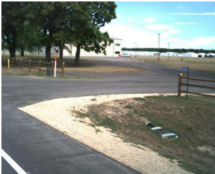
Figure 20.2 Good Parallel Slope and Traversable Endwall
