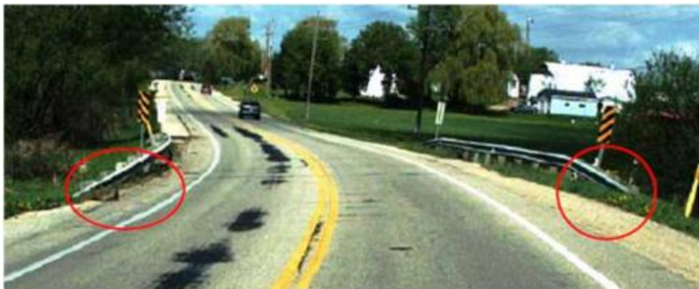
Figure 30.65 Downturned End Treatment
