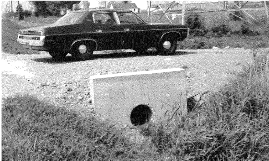
Figure 20.1 Parallel Slope Hazard
