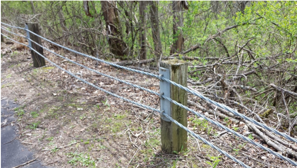
Figure 30.35 Strong Post Low-Tension Cable Barrier to be Replaced
