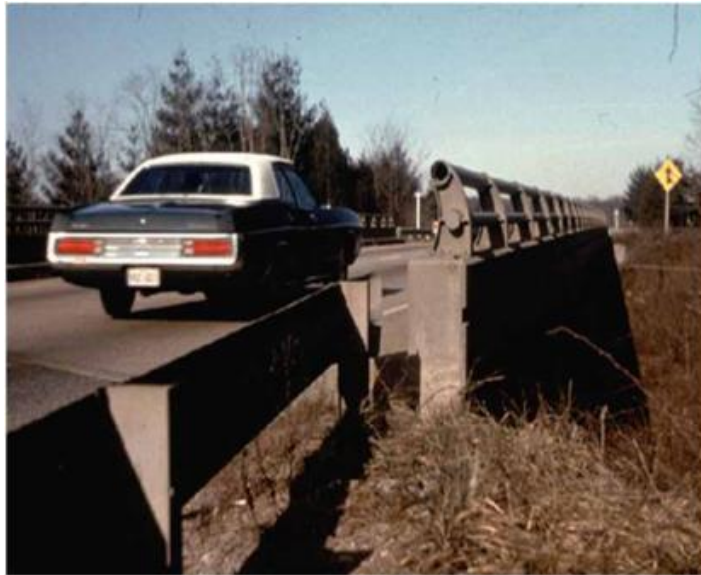
Figure 30.41 Unconnected Beam Guard xcix
