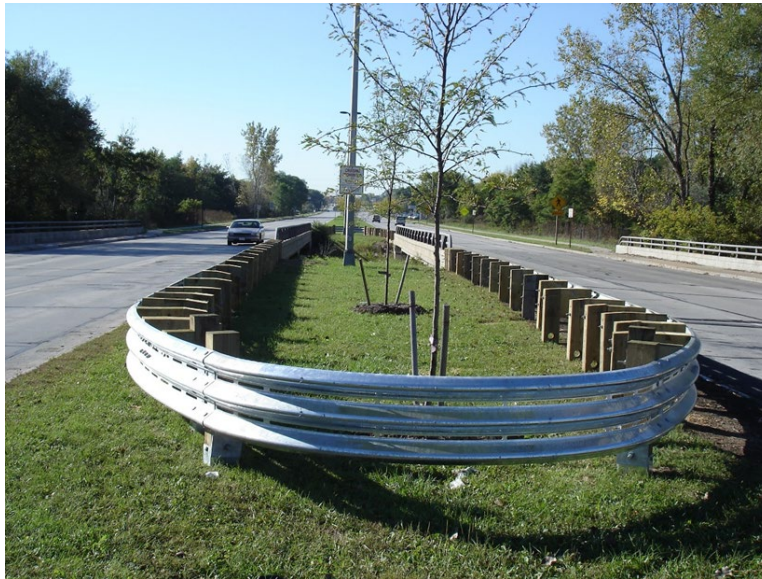
Figure 30.53 Trees placed within Bullnose
