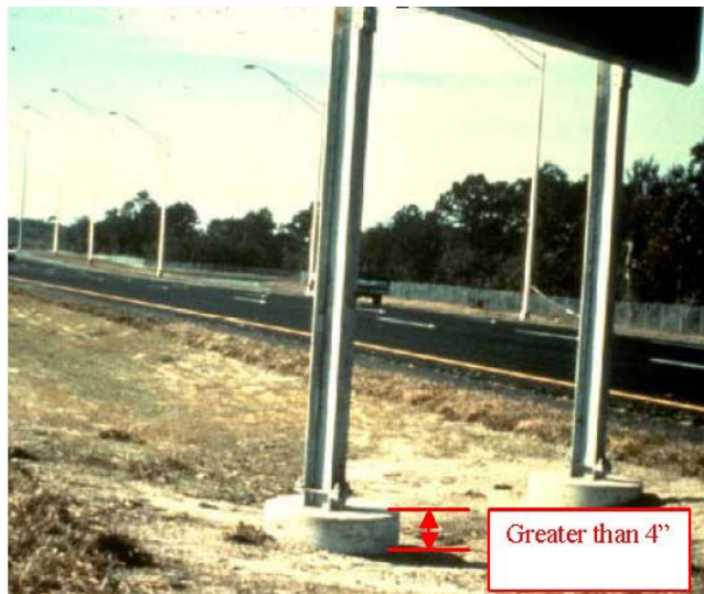
Figure 25.4 Improperly Installed Concrete Footing 3
