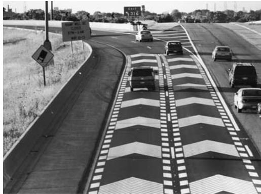
Chevron pavement markings help prevent truck tip-overs on a ramp of the Mitchell Interchange in Milwaukee.
