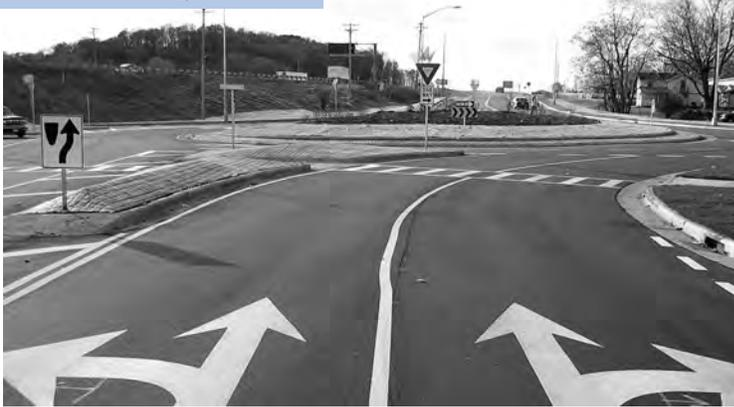
**WIS 30 and Thompson Drive in Madison.** Single white pavement marking line separating the two entry lanes. A large truck can straddle the lanes at entry. Truckers generally try to protect the right side of their vehicles by not allowing other autos from driving on their right (blind) side.
