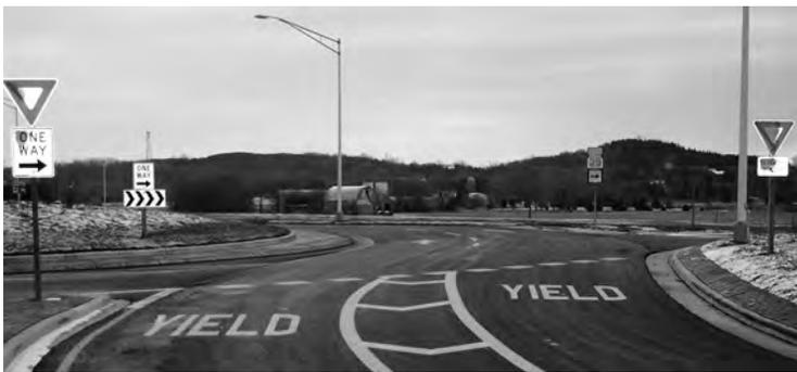
**STH 35 and Hanley Road near Hudson.** Double white pavement marking lines separating the two entry lanes. A large truck can stay in its lane when approaching.
