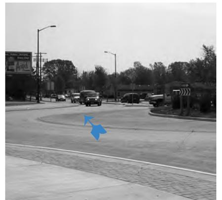
Roundabout at STH 64/STH 180 with wide truck apron to accommodate oversize-overweight vehicles.
