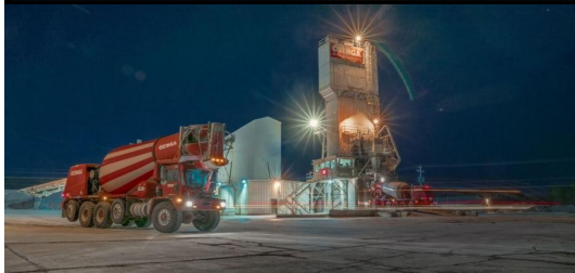
Concrete Batch Plant
