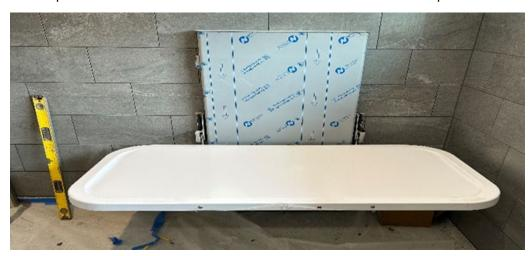
Contractors are actively building the new safety rest area along I-90 westbound near Sparta. The adult changing tables are being installed in separate family-assisted restrooms in the building.
