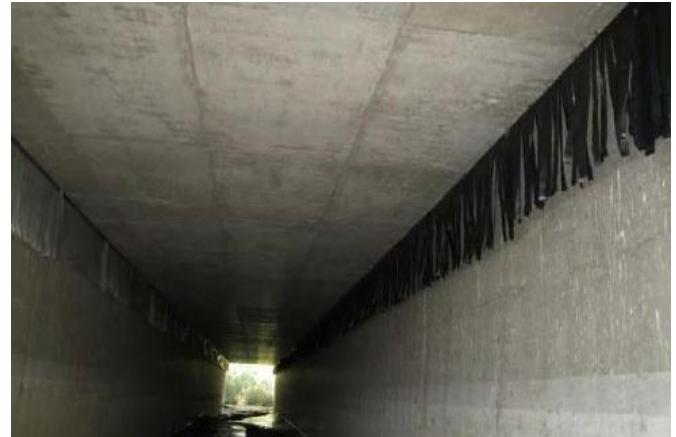
Flexible strip curtains in a concrete box culvert
