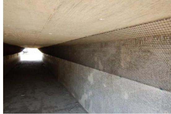
Properly installed culvert corner netting (TxDOT)
