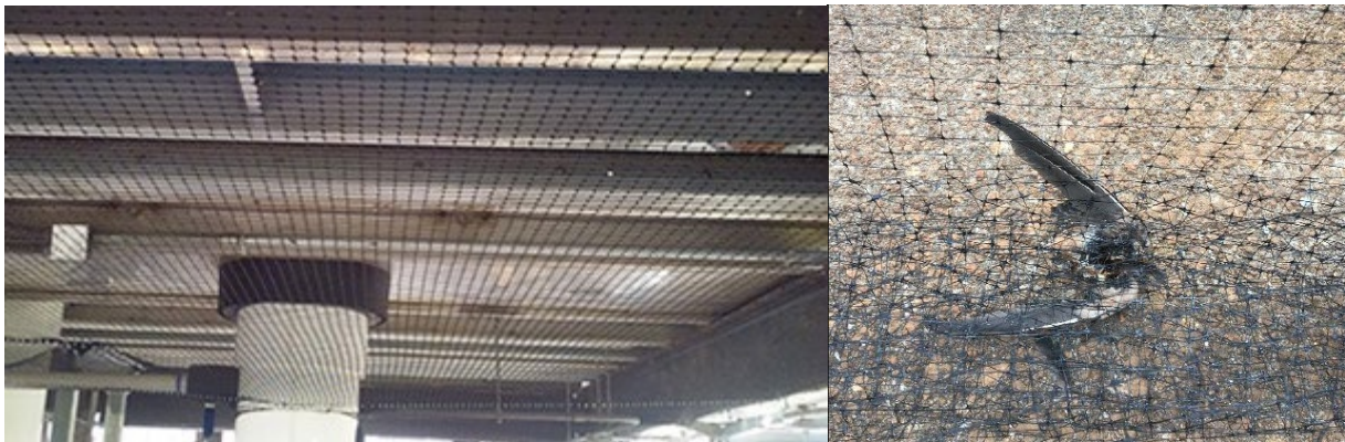
Left: properly installed bridge netting (netting.com) Right: bird mortality from net entanglement (GDOT)
