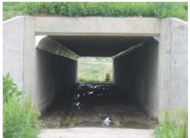
Properly installed corner slopes on a box culvert (GDOT)
