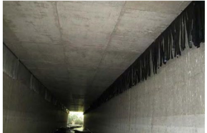
Flexible strip curtains in a concrete box culvert (Tate 2010)
