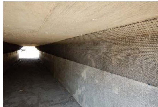
Properly installed culvert corner netting (TxDOT)
