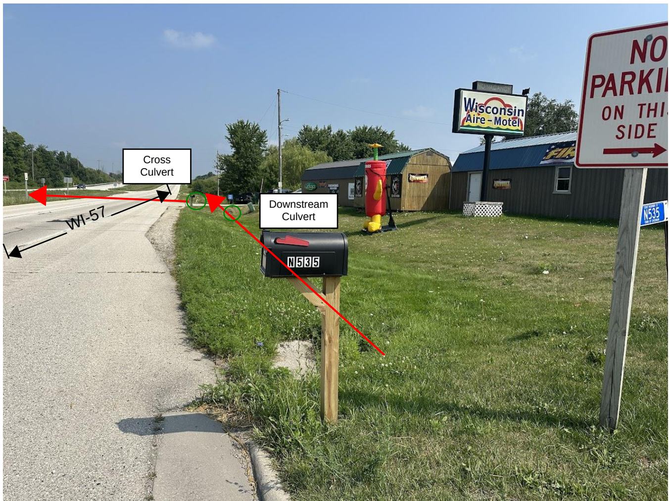
Photo taken facing north next to the Wisconsin Aire-Motel. Runoff is conveyed through the downstream culvert, with a portion of the flow diverted west into the cross culvert along WI-57.
