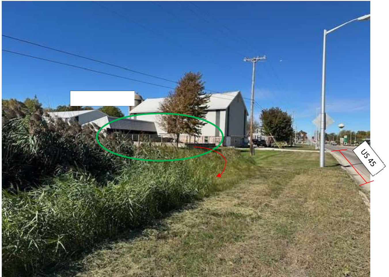
Drainage towards vegetated ditch
