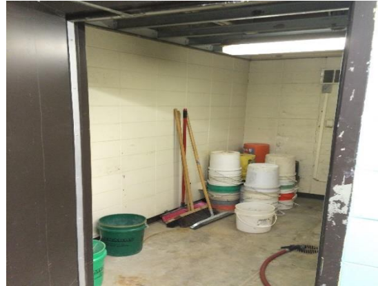
Vacant Concrete Cure Room
