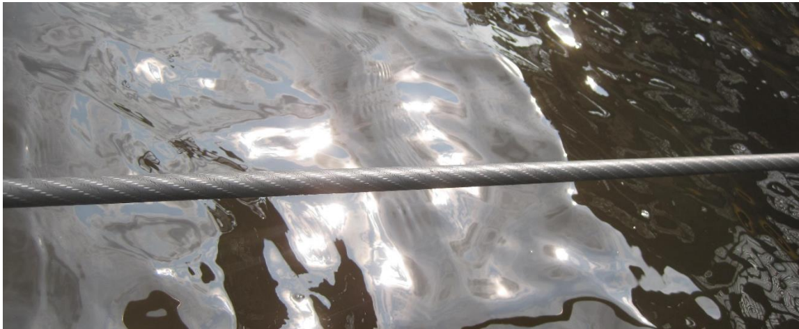
Figure 12: Drive Cable, Marine growth near South landing
