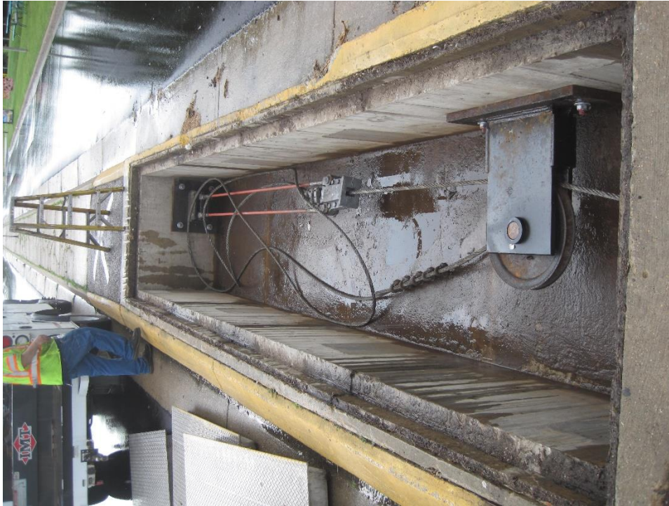
Figure 13: Drive Cable Anchorage, South Landing
