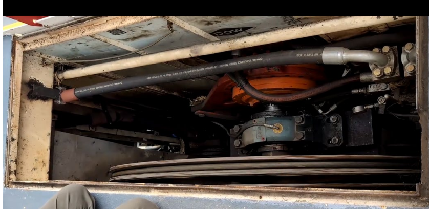
Figure 2: Routine Cable Inspection
