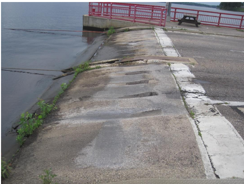
Figure 6: Vessel Ramp, North Landing
