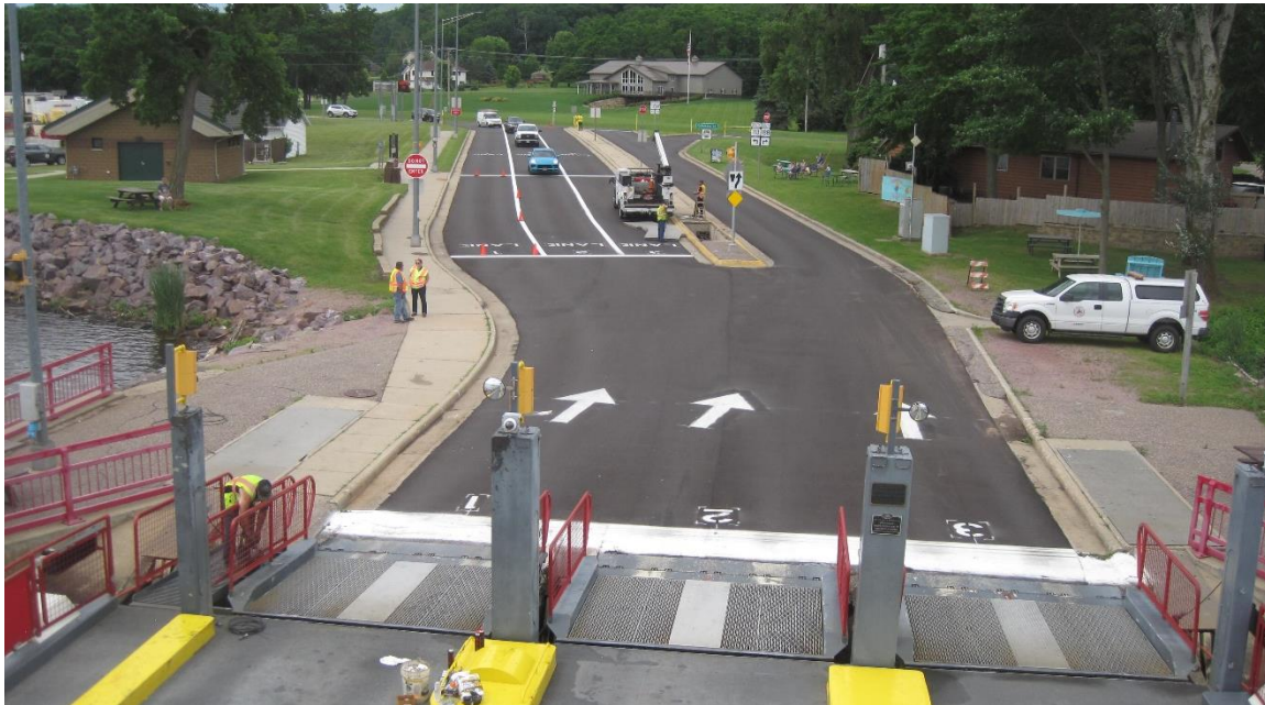
Figure 10: Upland Paving, South Landing
