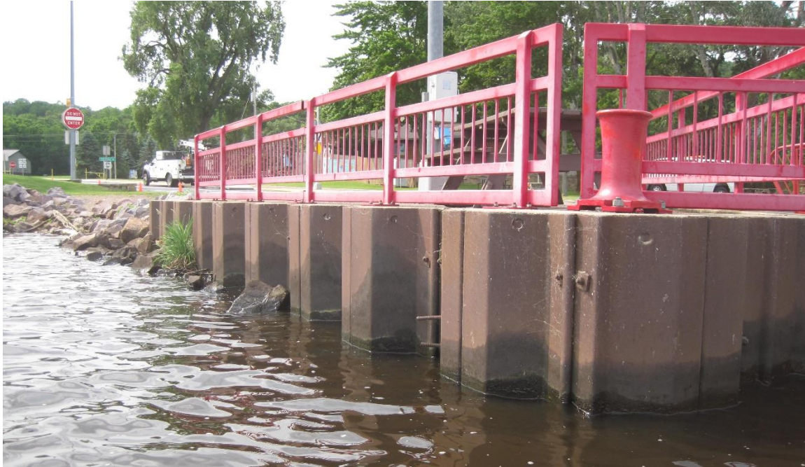
Figure 1: Steel Sheet Piling, Typical Conditions, SE Corner Shown
