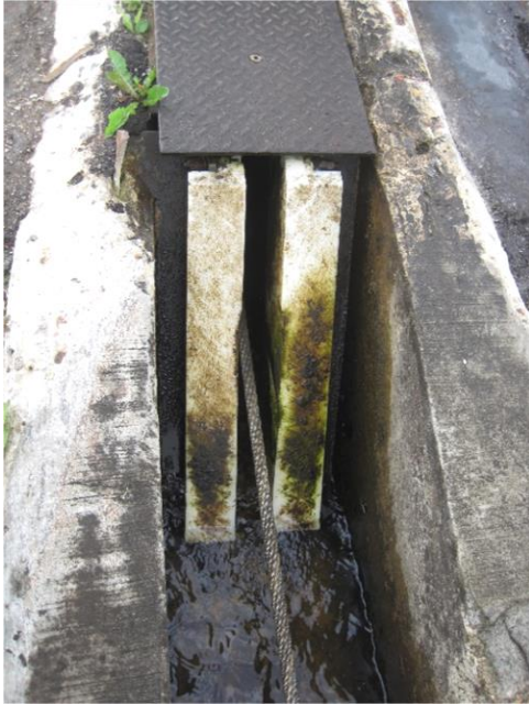
Figure 18: Uneven Wear of drive cable guides at trough exit locations, south (left)
