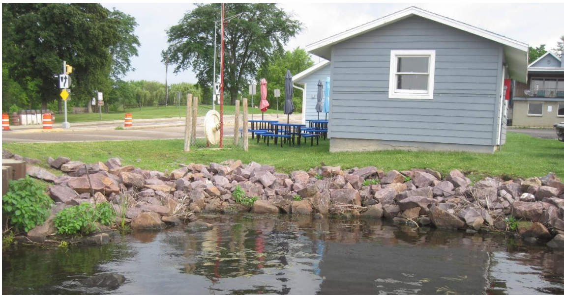
Figure 4: Riprap slope, Typical Conditions, NE Corner shown
