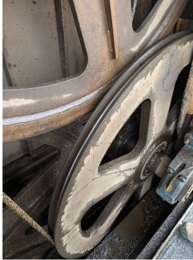
Figure 4: Sheaves, Older Construction Top, Newer Construction Below
