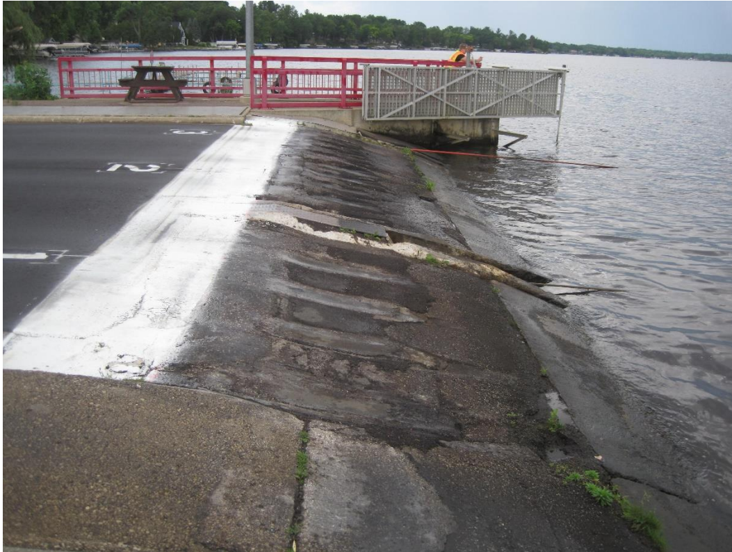
Figure 5: Vessel Ramp, South Landing
