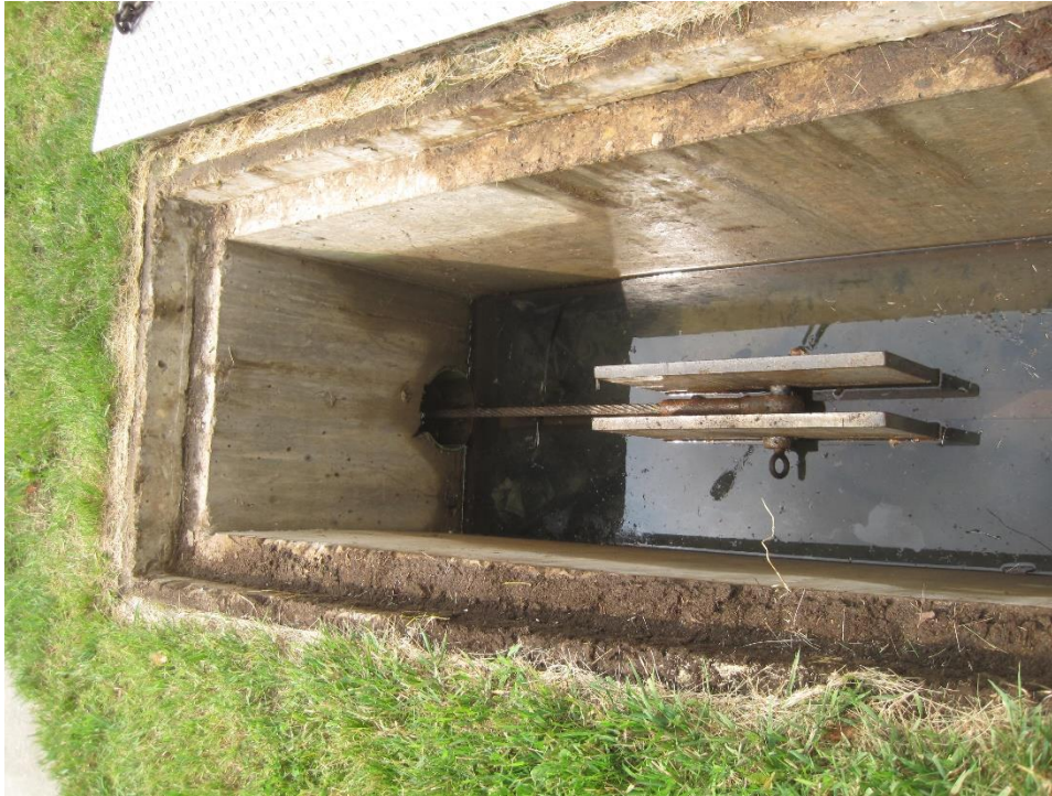
Figure 15: North drive cable anchor pit; standing water
