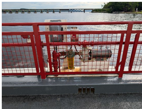
Figure 6: Fire Pump
