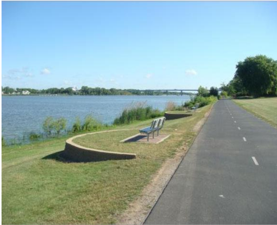
Photo: Fox River Trail in Green Bay, WI. Source: Matt Clark, National Transportation Alternatives Clearinghouse / www.ta-clearinghouse.info .
