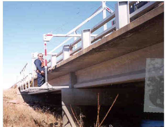
Class 9118 Scaffolding w/ electric hoist
