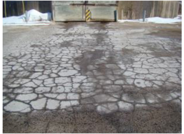
Severe cracking over entire apron (Bad - 5 total points)
