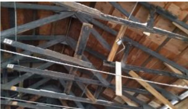
Ceiling trusses are damaged and not repaired (Poor - 40 total points)
