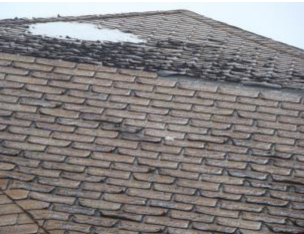
Weathered shingles-curved/missing (Poor - 40 total points)
