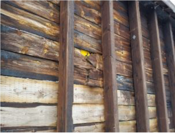
Cracked walls (Poor - 28 total points)
