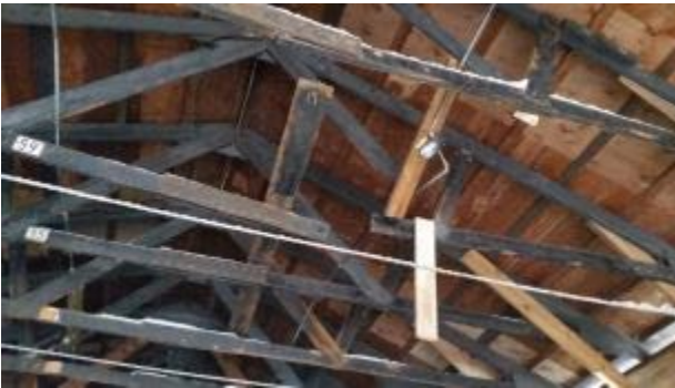
Ceiling trusses are damaged and unrepaired (Poor - 40 total points)
