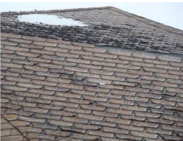
Weathered shingles-curved/missing (Poor - 40 total points)
