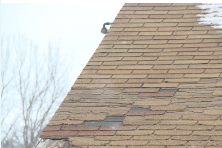
"Out of compliance" - salt shed in need of a new roof
