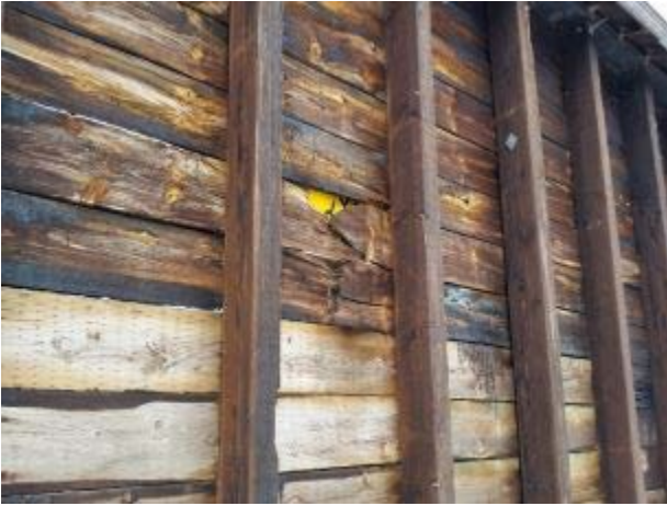
Cracked walls (Poor - 28 total points)
