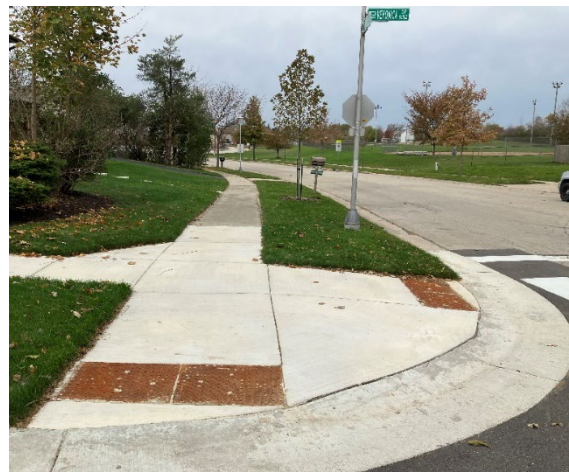
Figure 4.5 Curb Ramp - Oak Creek
