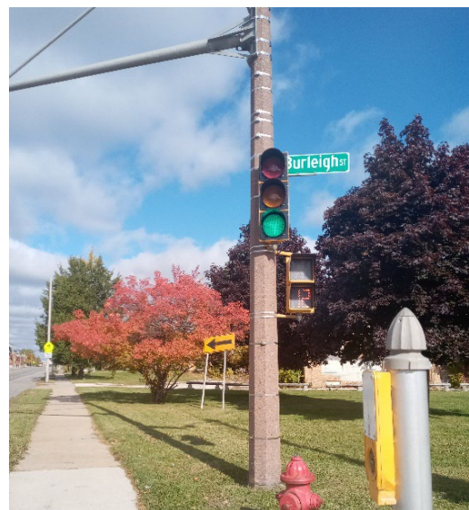
Figure 5.3 Traffic Lights – Milwaukee
