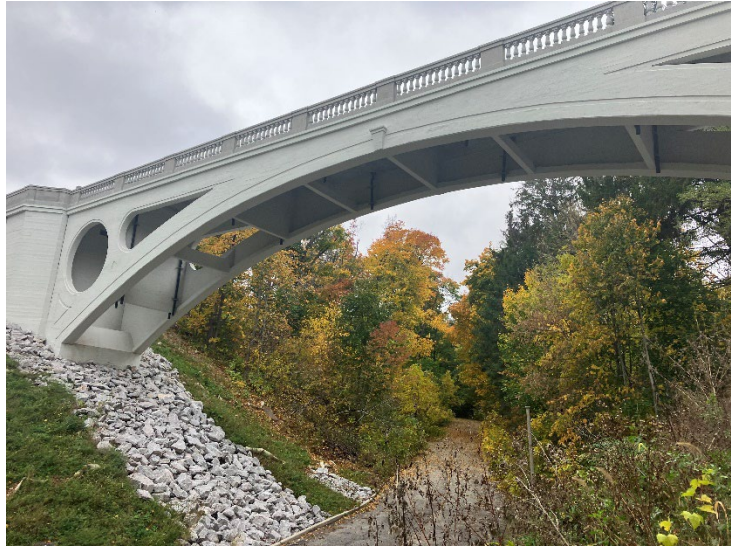
Figure 4.2 Lake Park Ravine Bridge - Milwaukee
