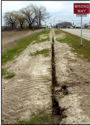
Figure 4: Examples of Improper ROW Restoration
