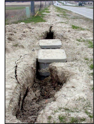
Figure 4: Examples of Improper ROW Restoration
