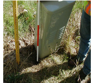
Figure 1. Pedestal too close to ROW pin.
