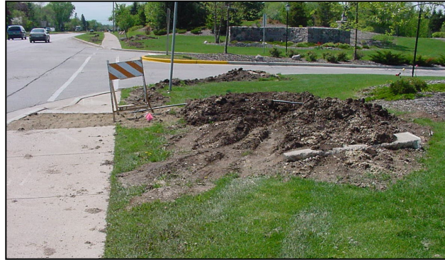
Figure 4: Examples of Improper ROW Restoration
