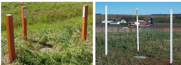
Figure 4. Orange guard or white witness posts surround a typical geodetic control monument installation. Some monuments may have 1 or 2 posts.
