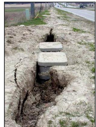
**Figure 3: Examples of Improper ROW Restoration**
