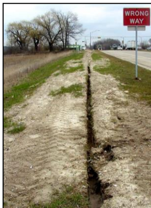
Figure 34: Examples of Improper ROW Restoration
