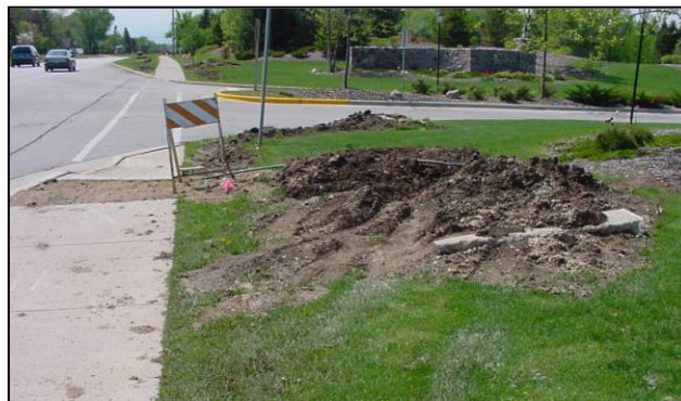
Figure 34: Examples of Improper ROW Restoration
