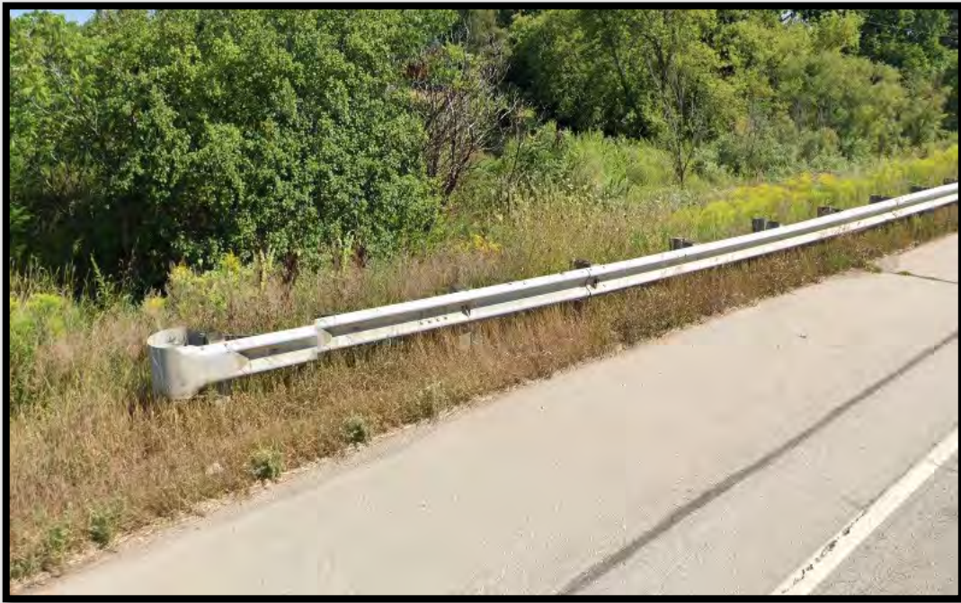
Existing beam guard along WIS 32/57
