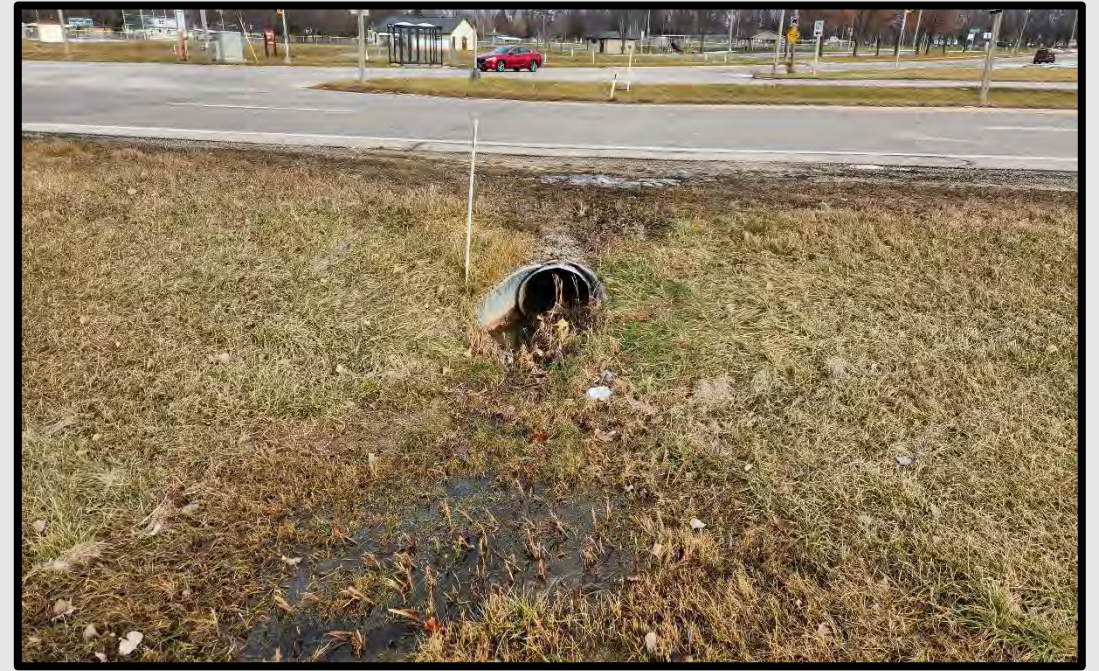
Existing culvert along WIS 32/57
