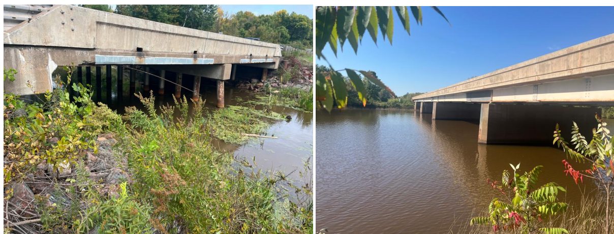
Figure 7 – B-02-006 over Kakagon Slough & B-02-005 over the Bad River main channel
