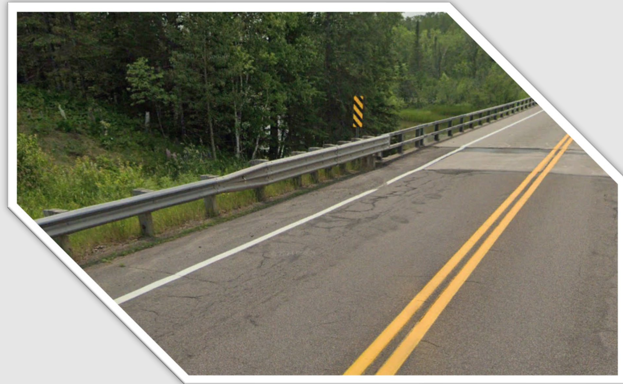
Iron River Bridge approach
