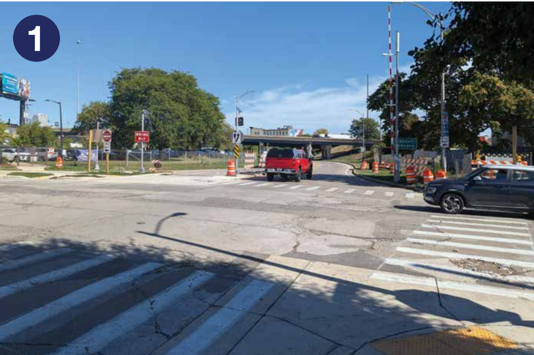
Entrance and exit ramps at 9th Street and Walker Street Rampas de entrada y salida en la calle 9th Street y la calle Walker Street
